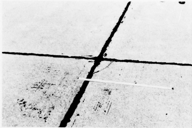
Figure A-135. Low Severity Corner Spall.
