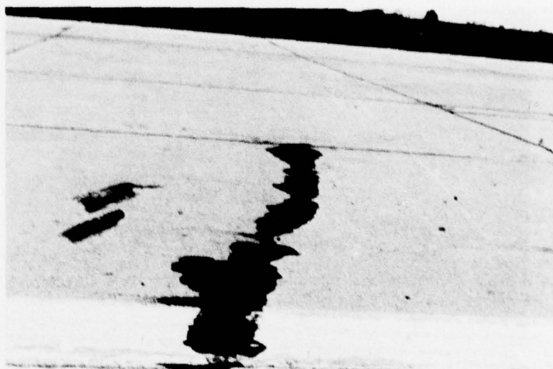
Figure A-83. Medium Severity Transverse Crack.
