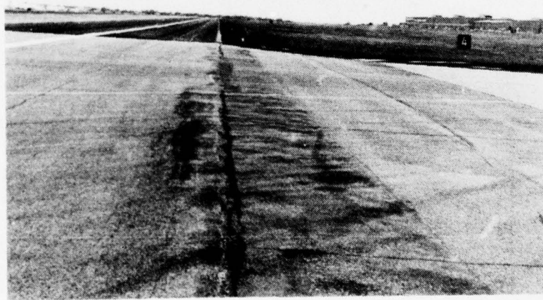
Figure A-63. This Photograph Shows a Shove of Low Severity on the Outside and Medium Severity in the Middle.
