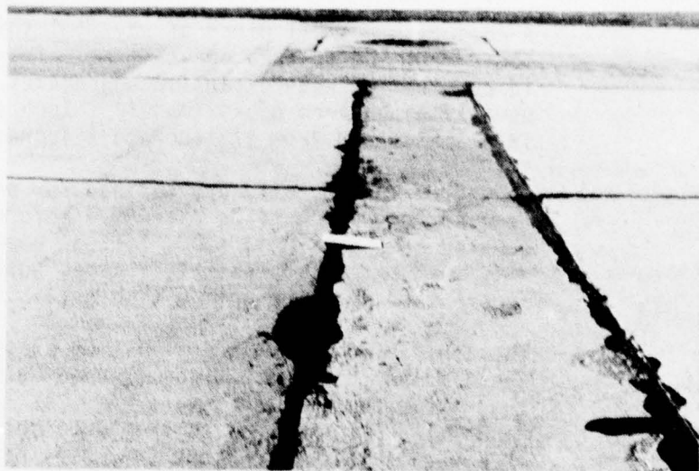
Figure A-104. Medium Severity Utility Cut.
