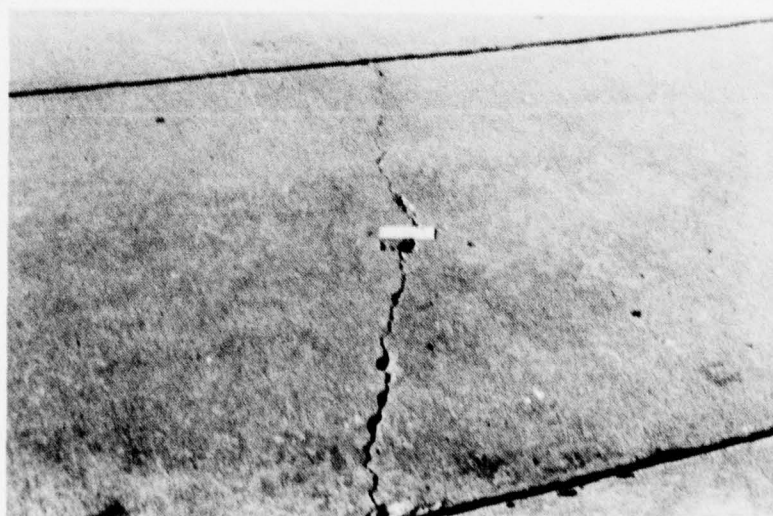
Figure A-84. Medium Severity Transverse Crack.
