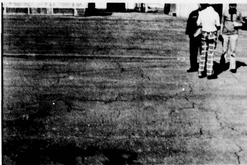
Figure A-13. Low Severity Block Cracking.
