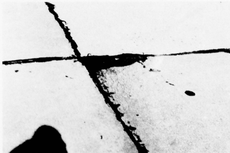
Figure A-88. Low Severity "D" Cracking.
