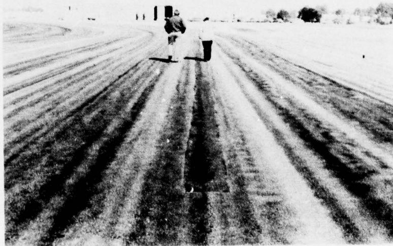
Figure A-46. Light Severity Patch.
