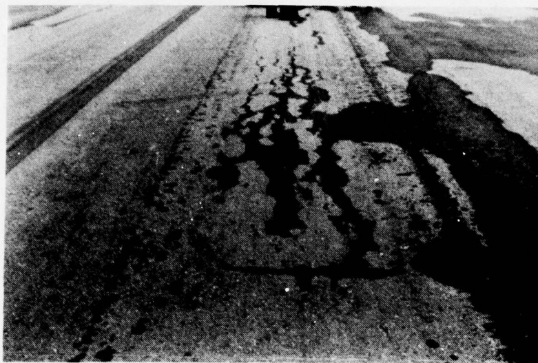
Figure A-3. Low Severity Alligator Cracking.
