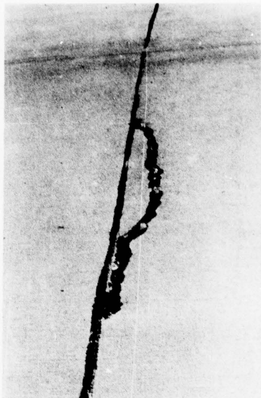
Figure A-130. Low Severity Joint Spall.
