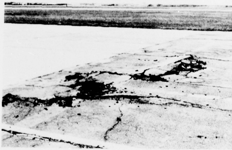
Figure A-64. High Severity Shoving.
