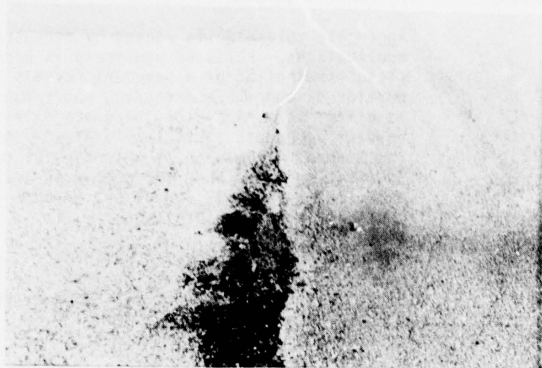
Figure A-49. Medium Severity Patch.
