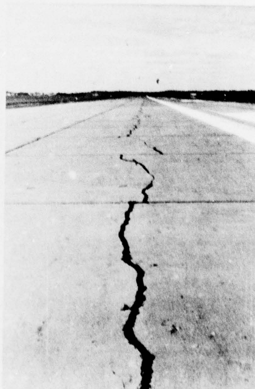
Figure A-80. Low Severity Filled Longitudinal Cracks.
