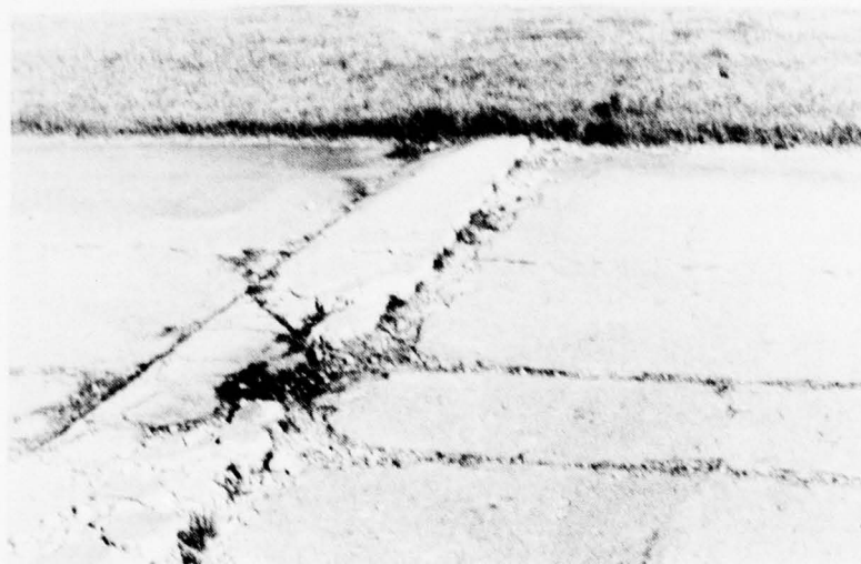
Figure A-73. High Severity Blow-Up.
