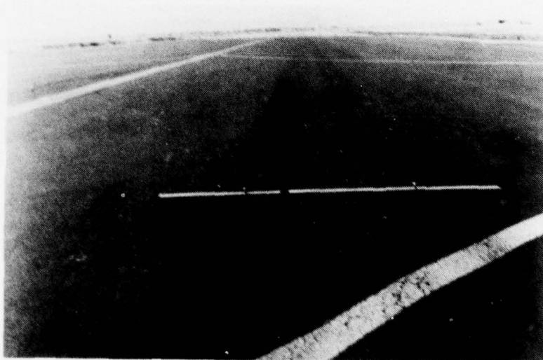
Figure A-62. High Severity Rutting. (Note Cracking and Upheaval on Sides of Rut.)
