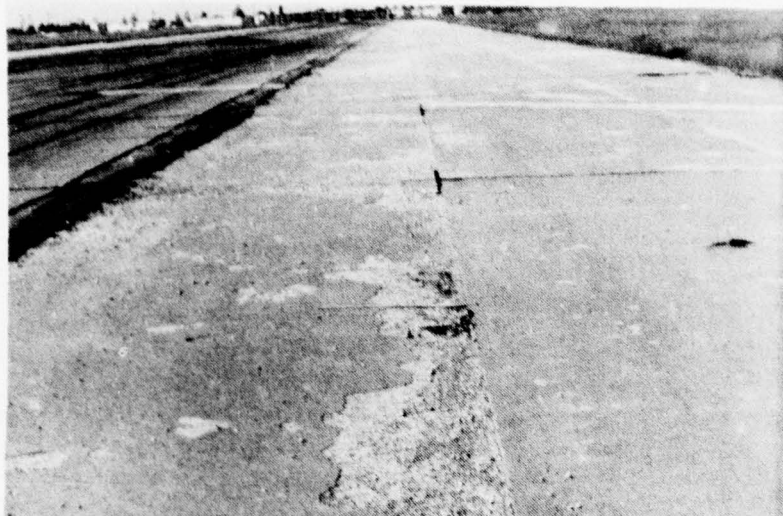
Figure A-113. High Severity Scaling.
