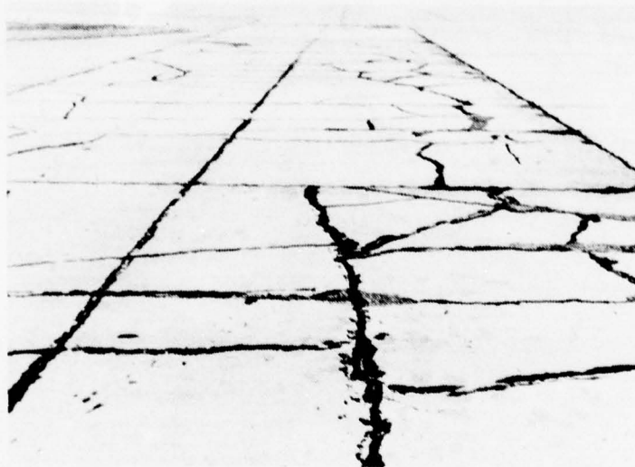
Figure A-124. Shattered Slab.
