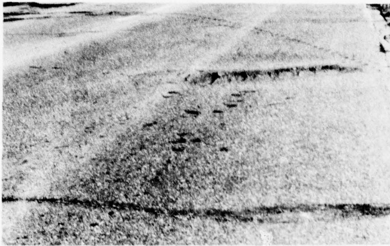
Figure A-69. High Severity Swell.
