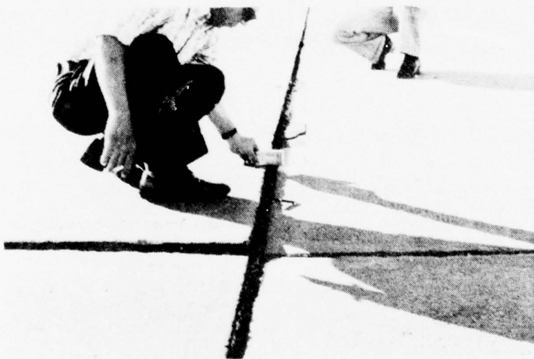
Figure A-119. High Severity Settlement.
