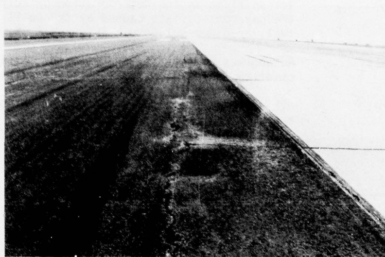
Figure A-42. Medium Severity Longitudinal Crack.
