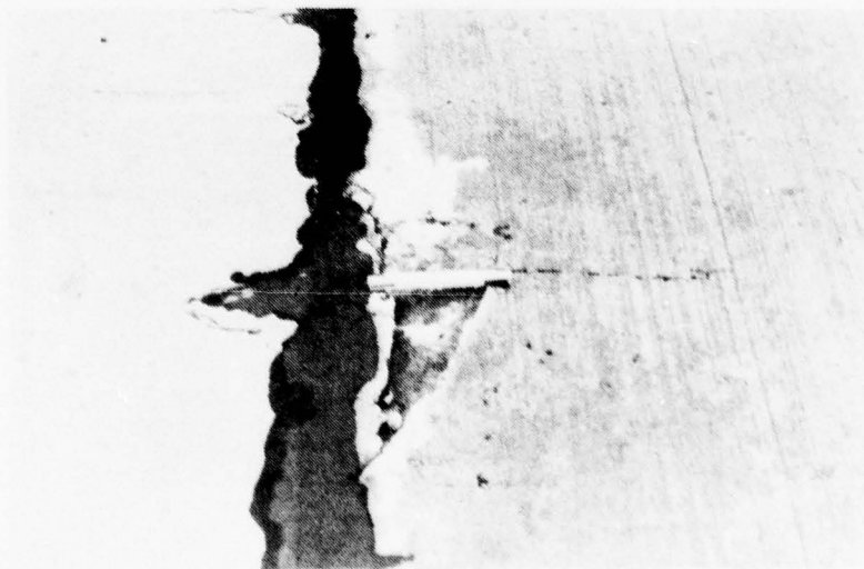
Figure A-131. Medium Severity Joint Spall.
