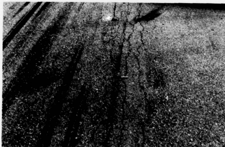
Figure A-4. Low Severity Alligator Cracking, Approaching Medium Severity.
