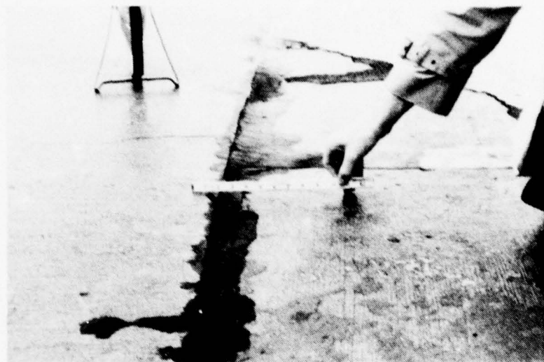
Figure A-117. Medium Severity Settlement on Apron ( > 1/2 Inch).
