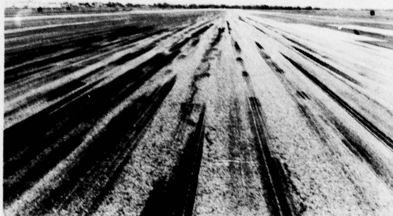
Figure A-39. Low Severity Longitudinal Cracks, Approaching Medium.
