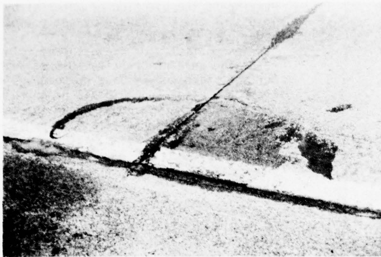
Figure A-107. Pumping. (Note Fine Material on Surface That Has Been Pumped Out, Causing Corner Break.)
