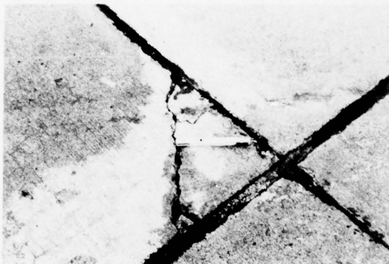
Figure A-137. Medium Severity Corner Spall.
