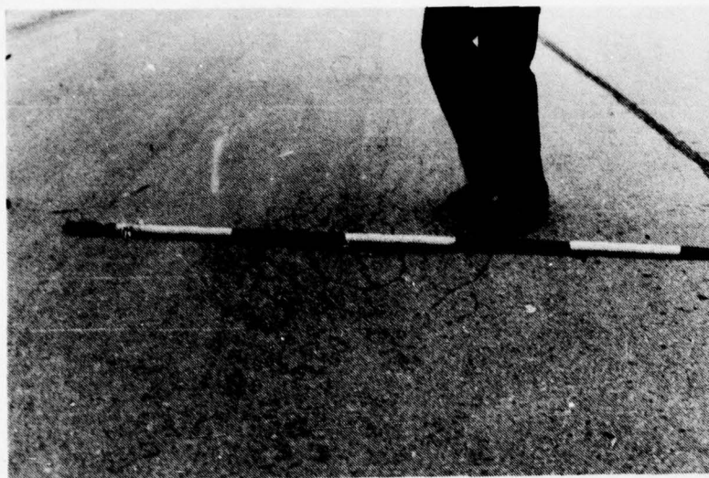
Figure A-5. Medium Severity Alligator Cracking. (Note the Depression Occurring With the Cracking.)
