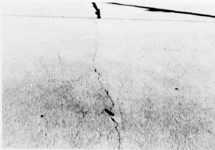
Figure A-79. Low Severity Longitudinal Crack.
