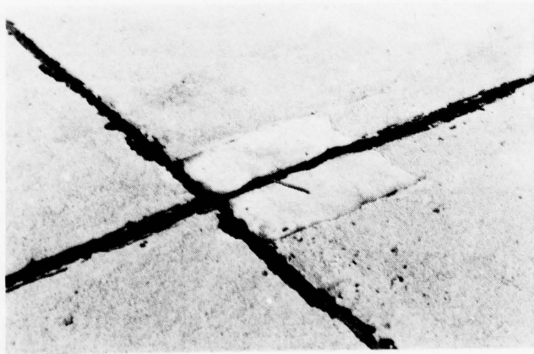
Figure A-96. Low Severity Small Patch.
