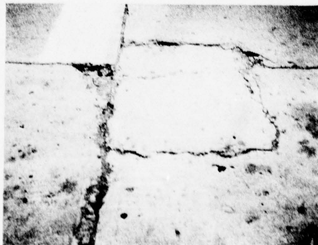
Figure A-105. High Severity Patch.
