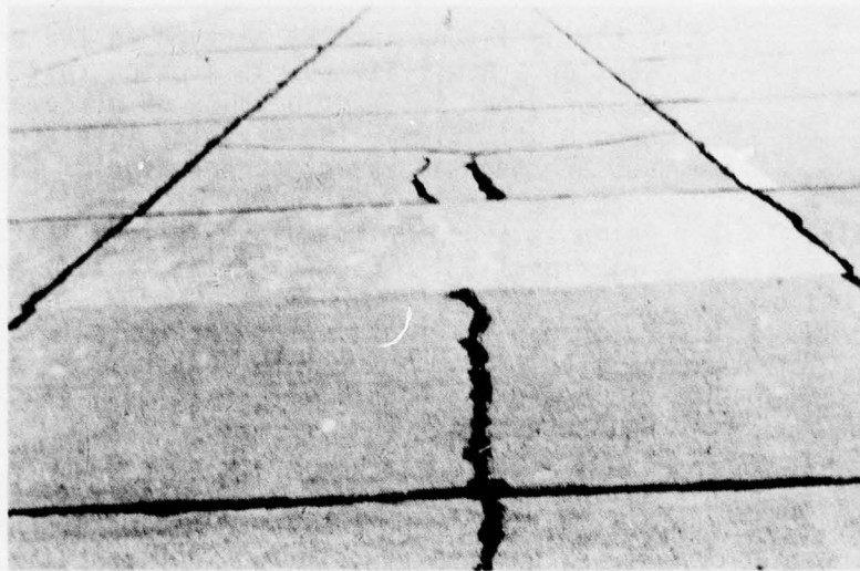
Figure A-102. Low Severity Patch.
