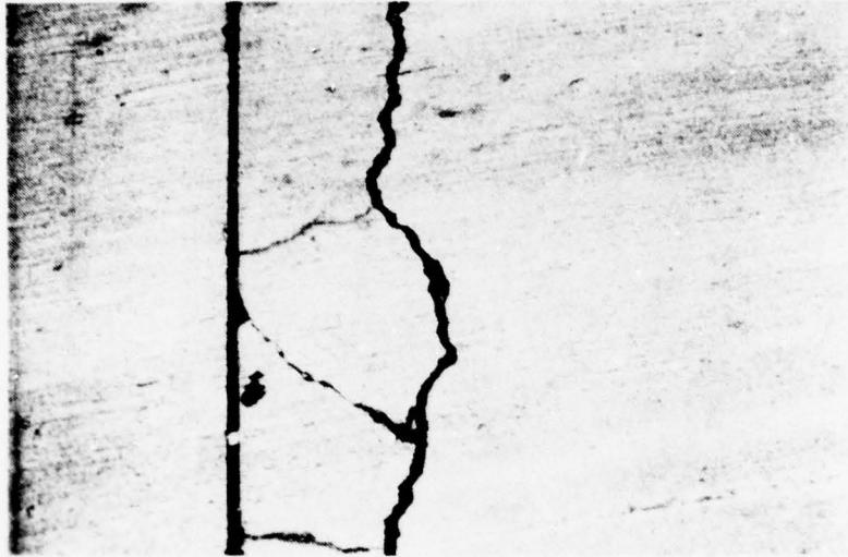
Figure A-132. Medium Severity Joint Spall.
