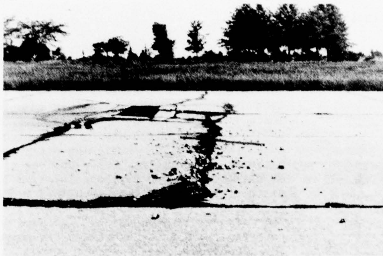
Figure A-71. Low Severity Blow-Up. (Note That This Would Only Be Considered Low Severity If the Shattering in the Foreground Was the Only Part Existing and the Foreign Material Removed.)
