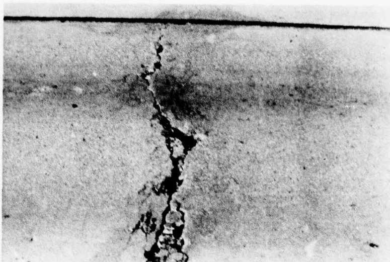
Figure A-85. High Severity Crack.
