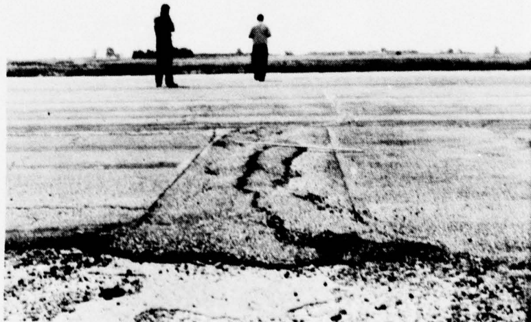
Figure A-50. High Severity Patch.
