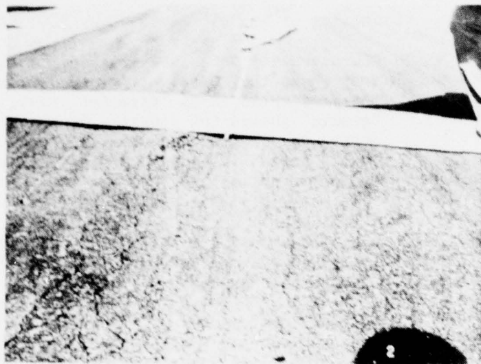
Figure A-61. High Severity Rutting. (Note Alligator Cracking Associated With Rutting.)
