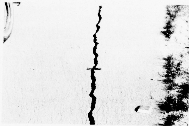
Figure A-87. High Severity Crack.
