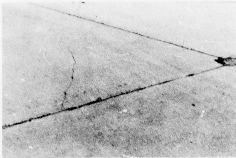
Figure A-81. Low Severity Diagonal Crack.
