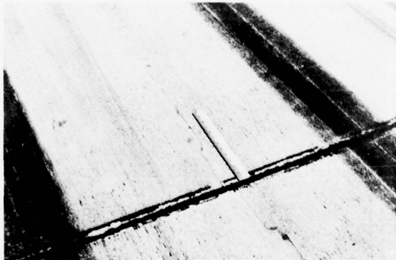
Figure A-125. Shrinkage Crack.
