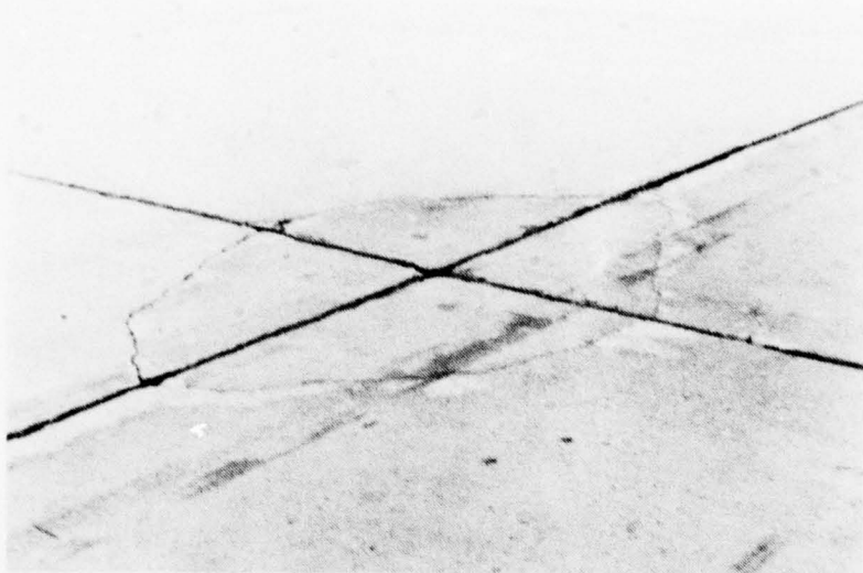
Figure A-74. Low Severity Corner Break.
