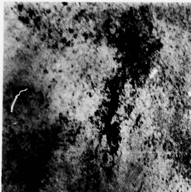
Figure A-55. Medium Severity Raveling/Weathering.
