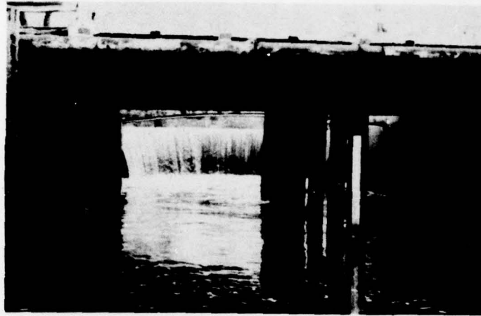
Photo 5 - Downstream view of the timber substructure of the bridge crossing the South Branch of the Metedeconk River; the spillway structure is in the background
