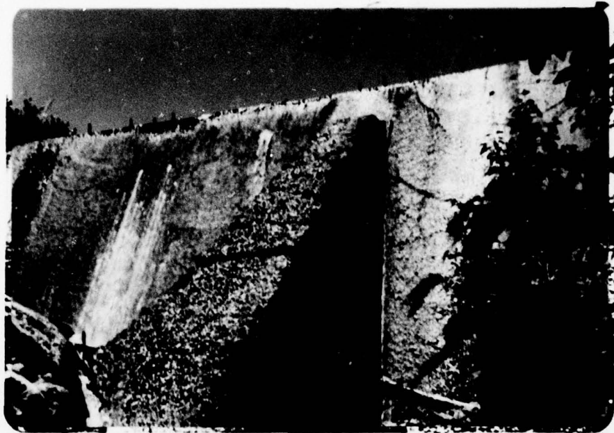
Central buttress pier at downstream face of spillway.
