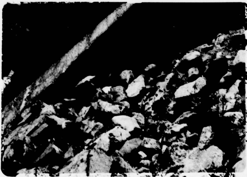
Erosion of riprap at spillway 19 June 1978 and left sidewall abutment.
