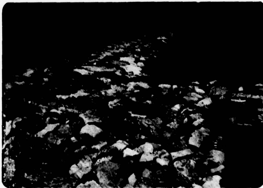
Upstream rip rap at right embankment. Looking west from intake structure.
