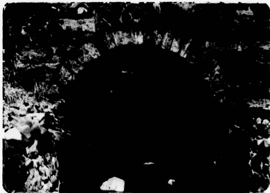
Culverts below road and Route 23 along spillway discharge canal looking downstream. Note boulder at end of culvert below road.
