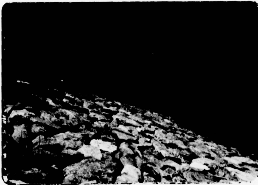
Upstream riprap at right embankment looking west from spillway.
