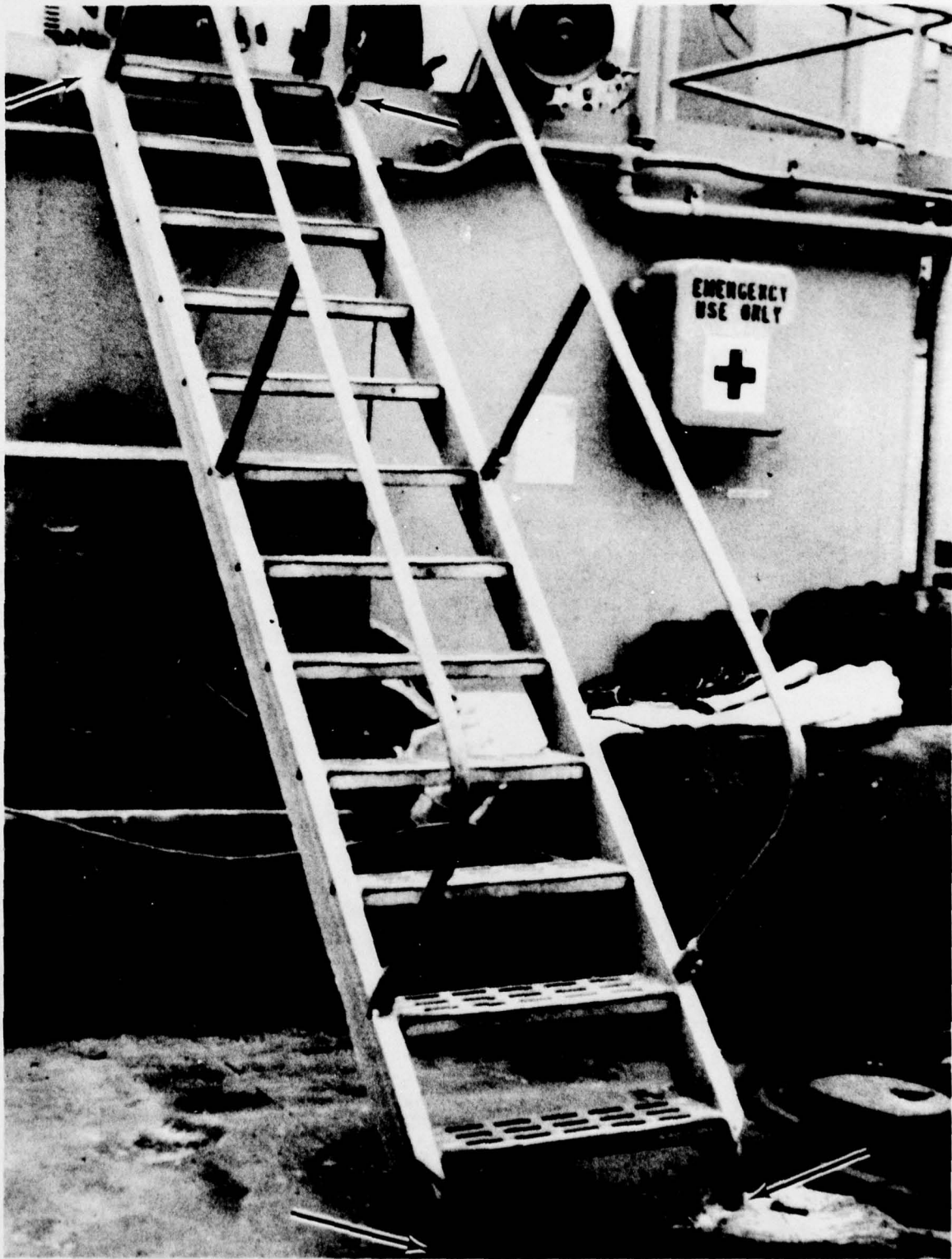
FIG. 11 INCLINED LADDER - TOGGLE BOLTS, WHERE LADDER MATES TO DECK, FORM NON-LINEAR JUNCTIONS THAT GENERATE IMI PRODUCTS
