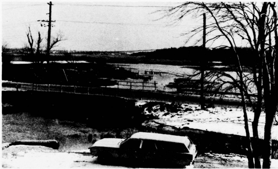
CHANNEL DOWNSTREAM OF SPILLWAY
