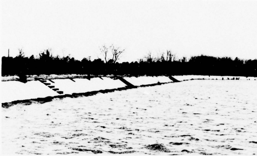
VIEW OF UPSTREAM FACE SHOWING AREAS OF SLOPE FAILURE
