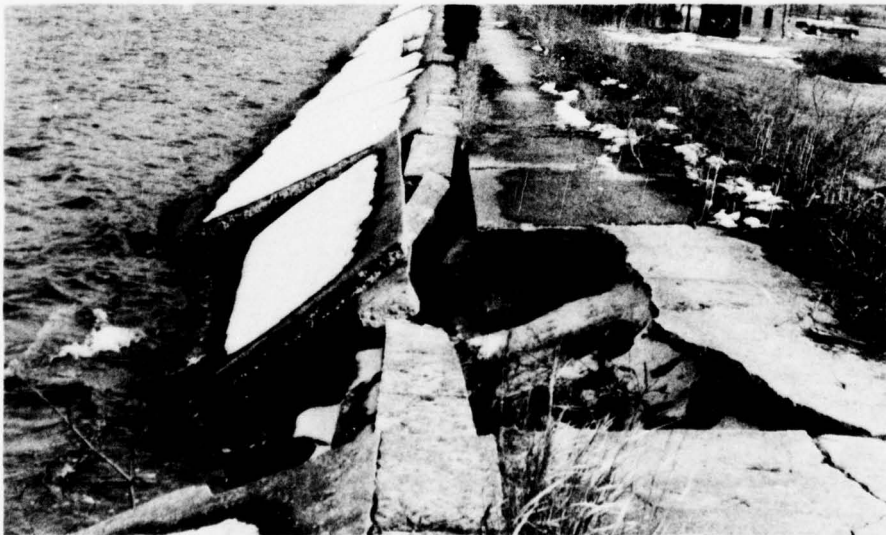
CLOSEUP OF UPSTREAM SLOPE FAILURE
