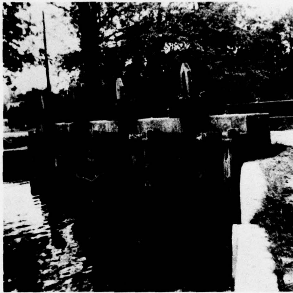
UPSTREAM FACE WITH GATES
