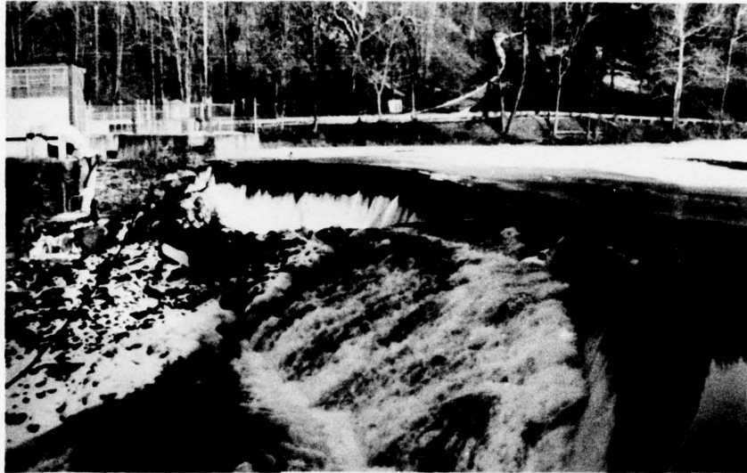
VIEW LOOKING TOWARD RIGHT BANK
