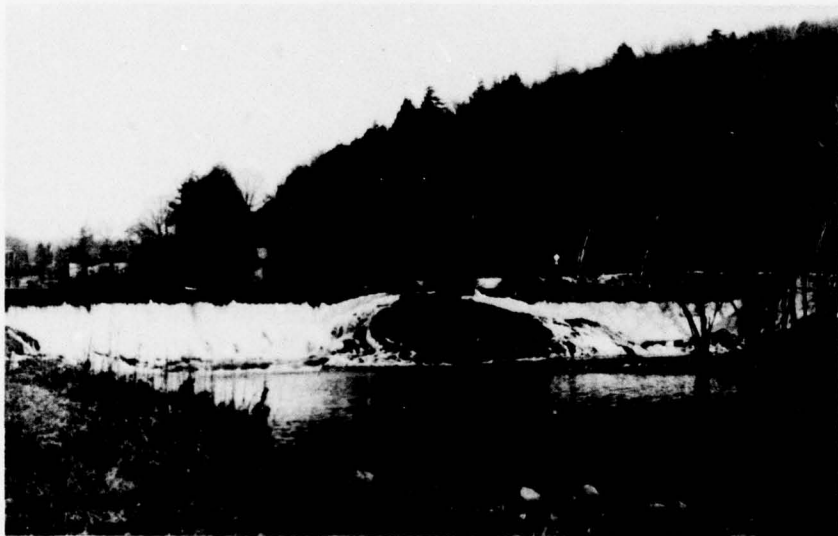
VIEW LOOKING UPSTREAM SHOWING ROCK OUTCROP AT CENTER AND EROSION OF HIGHWAY EMBANKMENT
