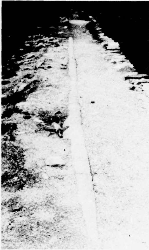
EXPOSED CONCRETE CORE
