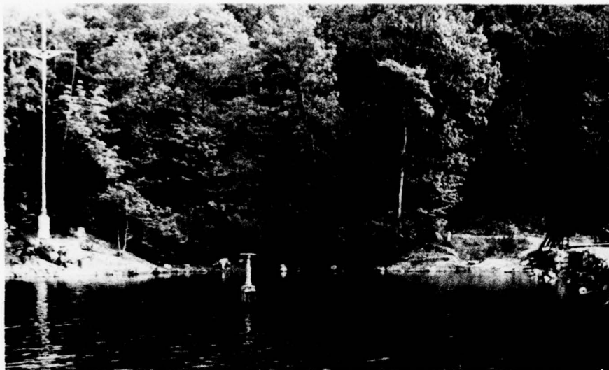
VIEW OF LEFT ABUTMENT NOTICE PEDESTAL FOR BOTTOM RELEASE GATE
