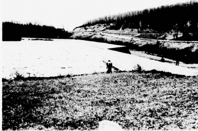
Photo 11 - River Wall - General view of River Wall looking upstream and north-west along the Pequannock River
