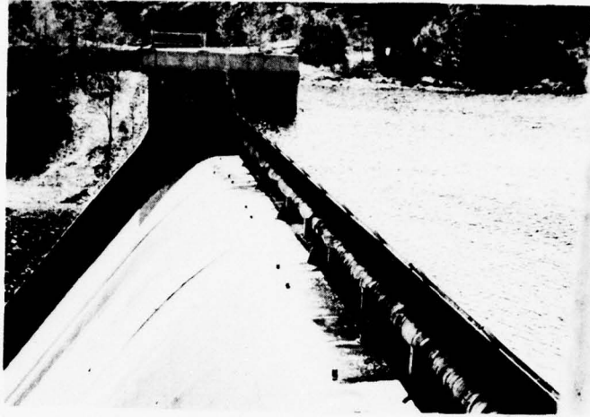
Photo 1 - View of spillway and bascule crest gate looking toward right abutment
