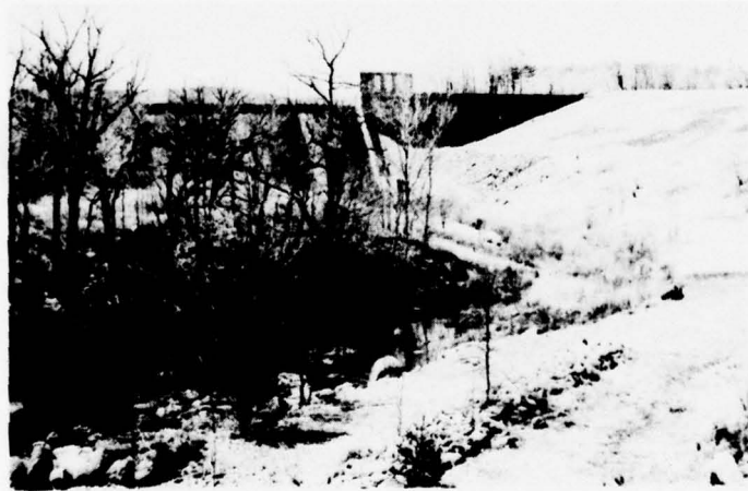
Photo 20 - View of downstream channel below dam; stony invert, well defined overbank valley
