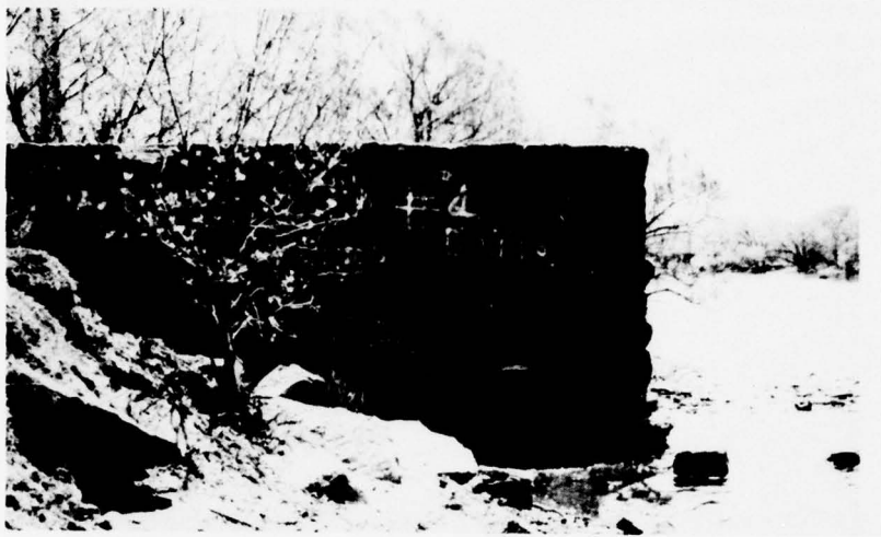
Photo 7 - View of left abutment from upstream side of dam
