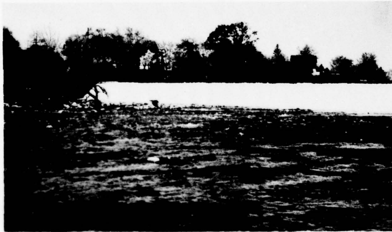
Photo 2 - View from downstream left bank looking toward right abutment
