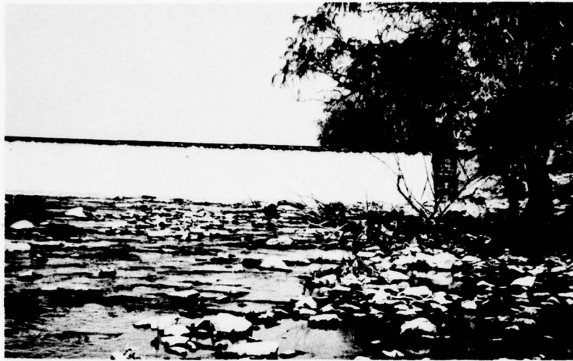
Photo 3 - View from downstream left bank at left abutment
