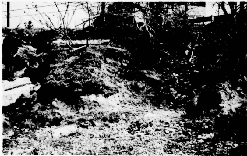
Photo 6 - Close-up view of left abutment area downstream of dam showing stream bank erosion caused by local street drainage overflow
