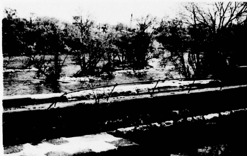
Photo 10 - View of Dundee Canal intake center wall (with railing) and cut down river wall acting as a sideweir beyond it
