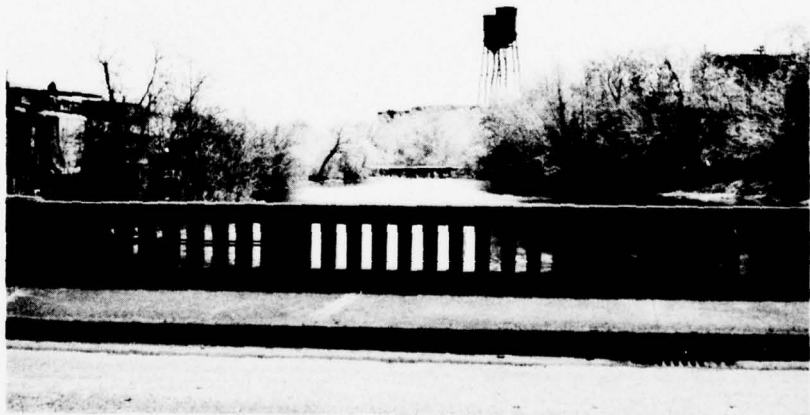
Photo 16 - View of Dundee Canal looking downstream of crossing at Ackerman Avenue, Clifton, NJ
