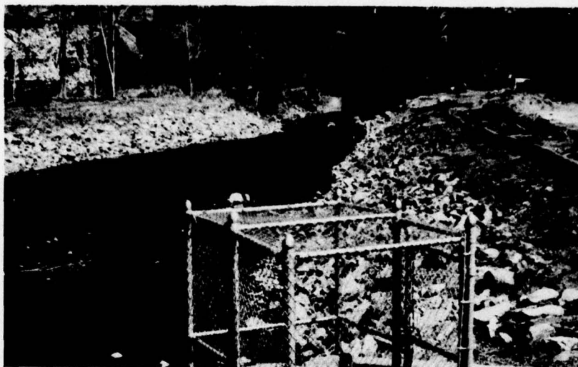
Photo 11 - View of downstream channel of Hohokus Brook; looking from right abutment area toward Hopper Avenue. The fenced enclosure in the foreground is to protect the 36-inch slide gate hoist stand on the low level outlet conduit.
