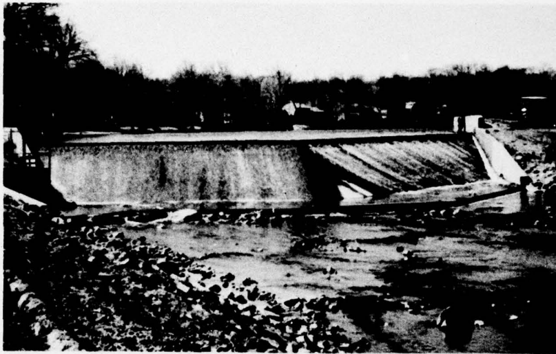
Photo 1 - View of dam from downstream; low level outlet facilities are on the left side of picture (right abutment)
