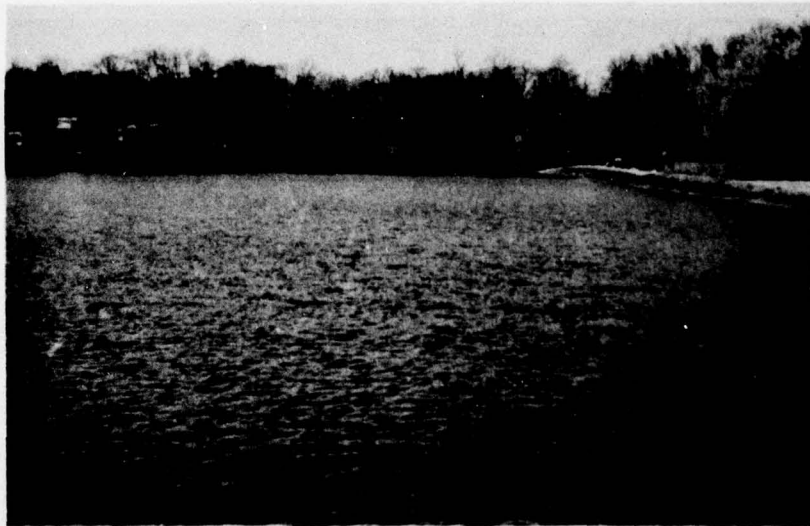
Photo 8 - View of White's Pond, looking toward the left shore line upstream of dam
