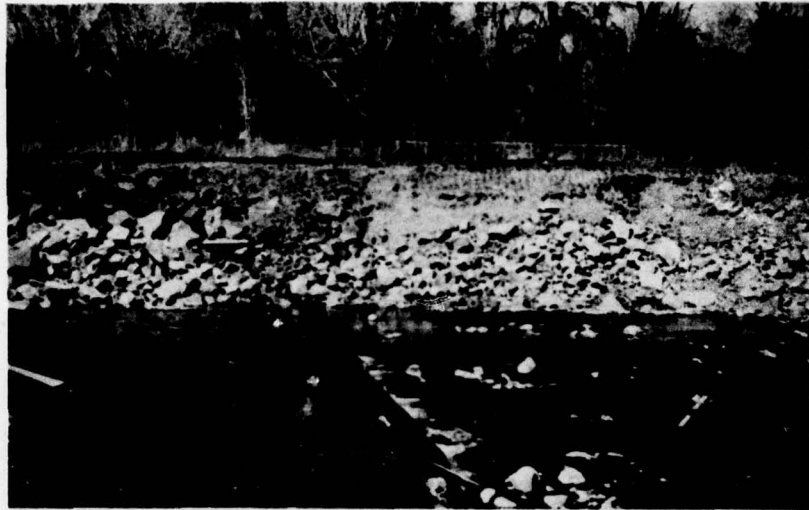
Photo 5 - View of damaged and slumping channel bank protection at the left channel bank caused by overtopping of the left abutment area by storm of November 7, 1977; the damaged area is at end of the stilling basin end sill visible in this picture
