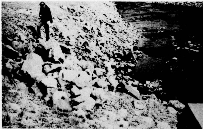
Photo 4 - View of eroded area behind the left abutment wingwall; abutment seepage observed in the area of crouching figure, approximately 20 ft. downstream of end of spillway wingwall
