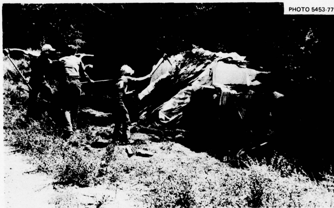
Fig. 4.30. Ridge-Pole Shelter nearing completion. The amount of earth required to cover the structure necessitates locating the shelter in an area where dirt can be easily excavated.
