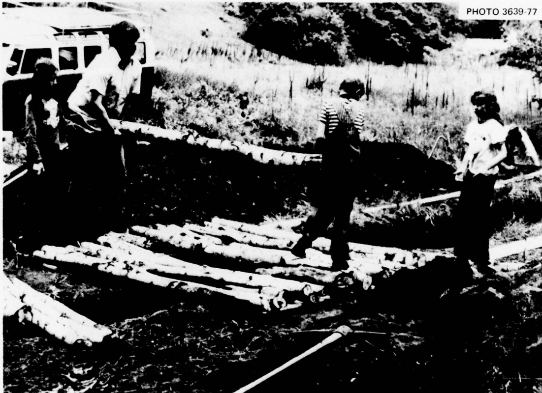
Fig. 4.12. Covering the trench with quaking aspen logs. These logs are indigenous to the area but are not as uniform in size nor as straight as lodgepole pine logs found in certain other areas. However, they did prove to be adequate for the task at hand.
