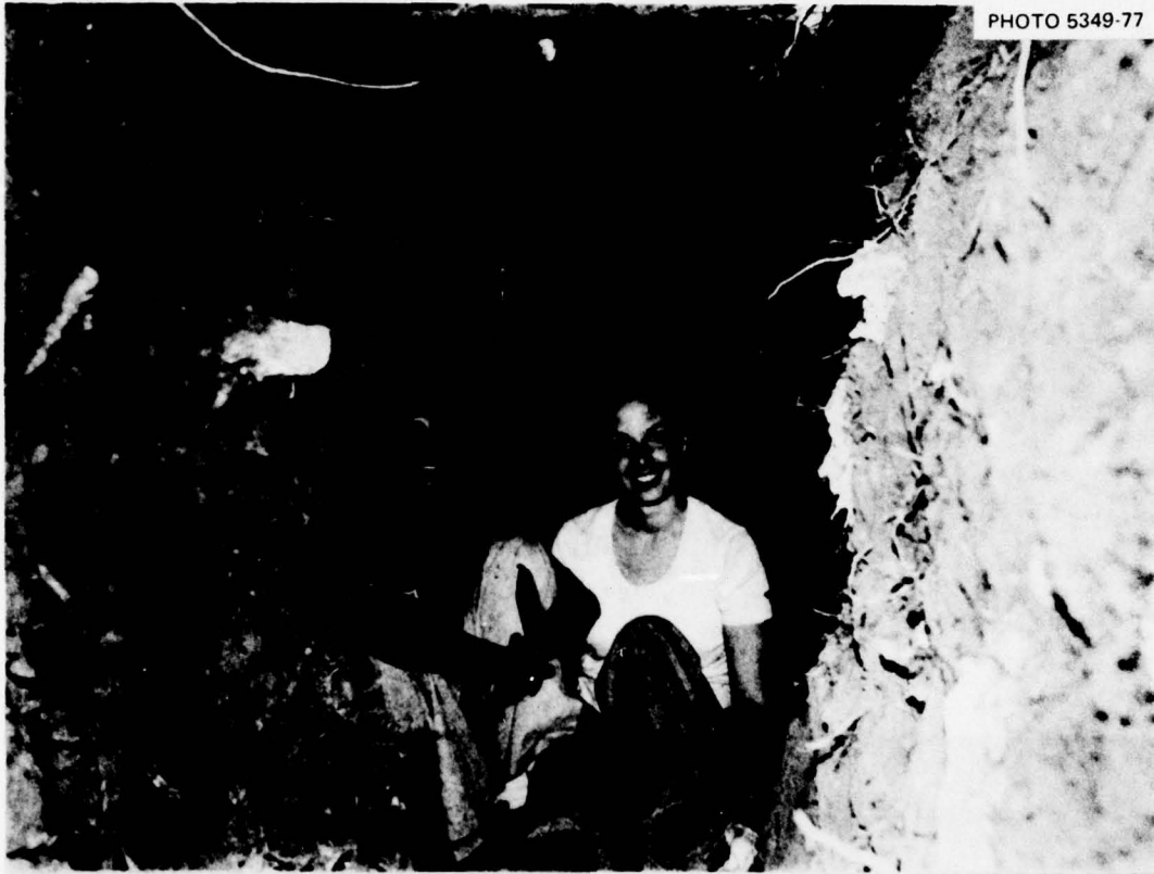
Fig. 4.3. Interior of Log-Covered Trench Shelter. (Note the large tree root system through which the trench was dug.)
