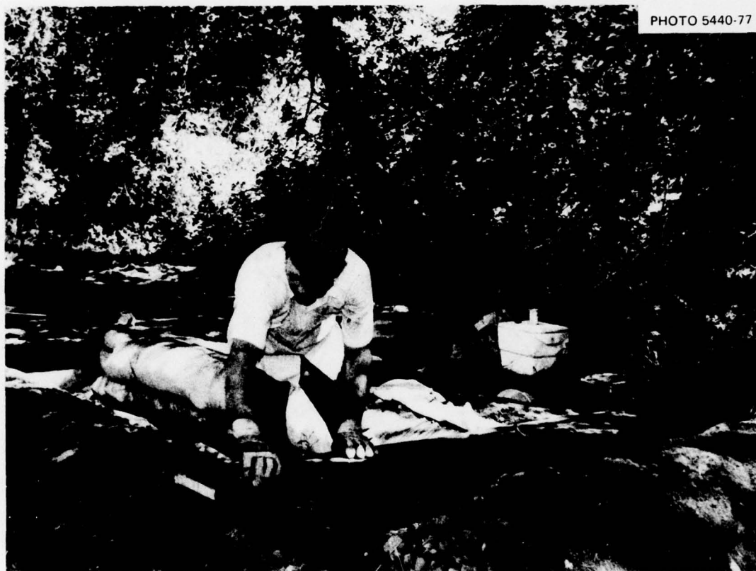
Fig. 4.19. Roofing on partly completed Aboveground Door-Covered Shelter. The last roofing door had not been placed.
