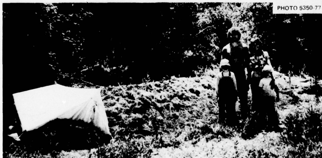
Fig. 4.5. Completed 4-person Log-Covered Trench Shelter. Flimsy canopy over entry is evidence of the need for better instructions and illustrations to enable an average American to make a stable canopy of specified height, with specified openings for adequate ventilation.
