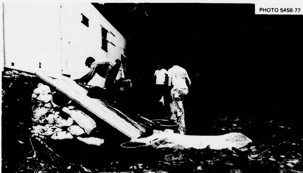
Fig. 4.34. End view of Tilt-up Door and Earth Shelter. It was a persistent challenge to keep dirt from sliding down the slanted doors.
