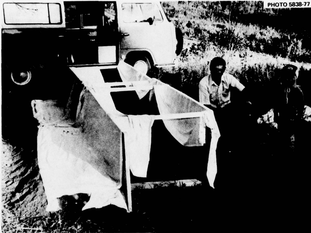
Fig. 4.18. Interior doors used for forms, preparatory to using bed-sheet fabric to make earth-roll walls.
