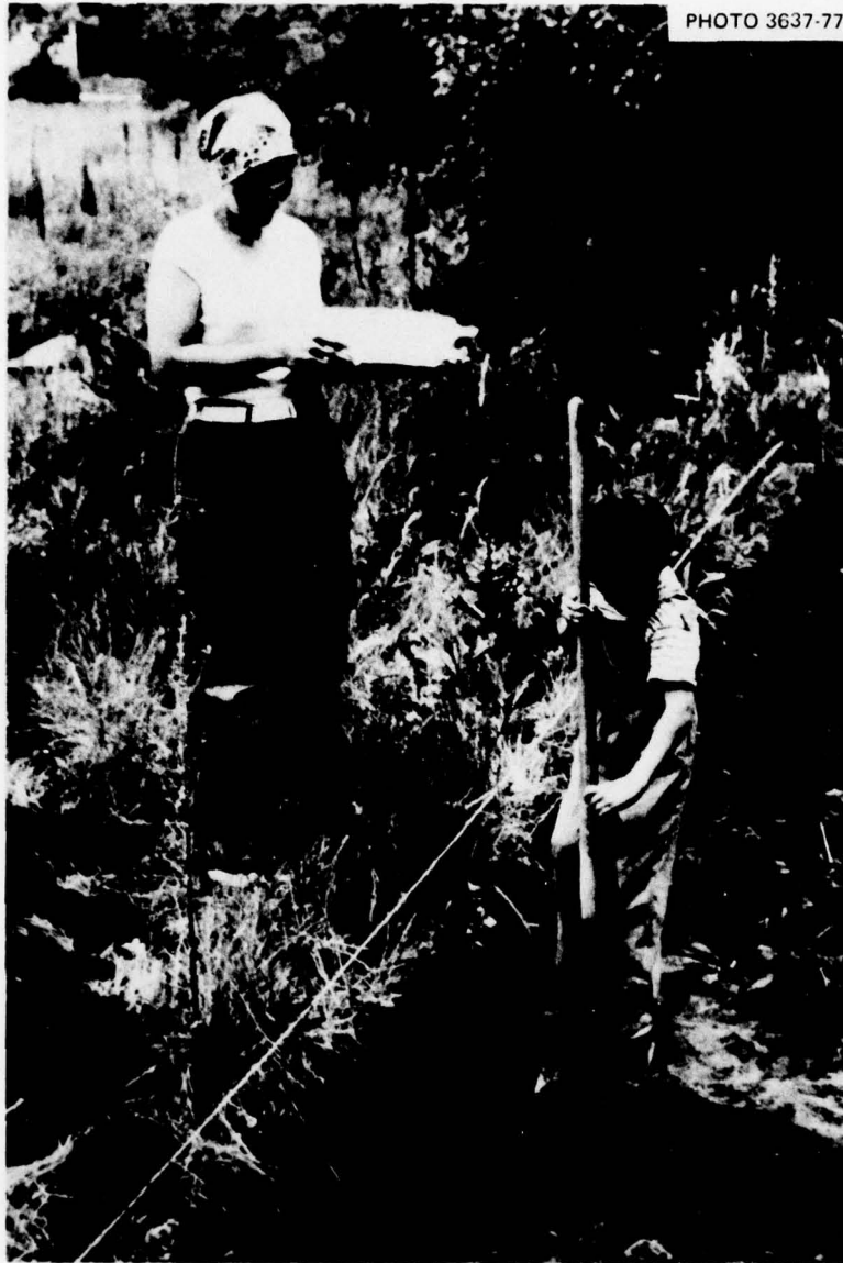
Fig. 4.6. The second Log-Covered Trench Shelter was constructed by a young family with six children under the age of 10. The children 5 and older helped in the construction. The father of this five-year-old showed him where and how to use a shovel in excavating the trench.
