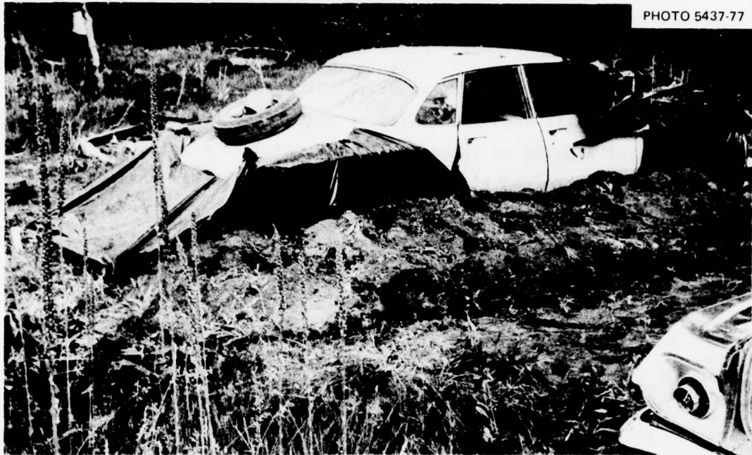
Fig. 4.16. Successfully completed Car-Over-Trench Shelter.
