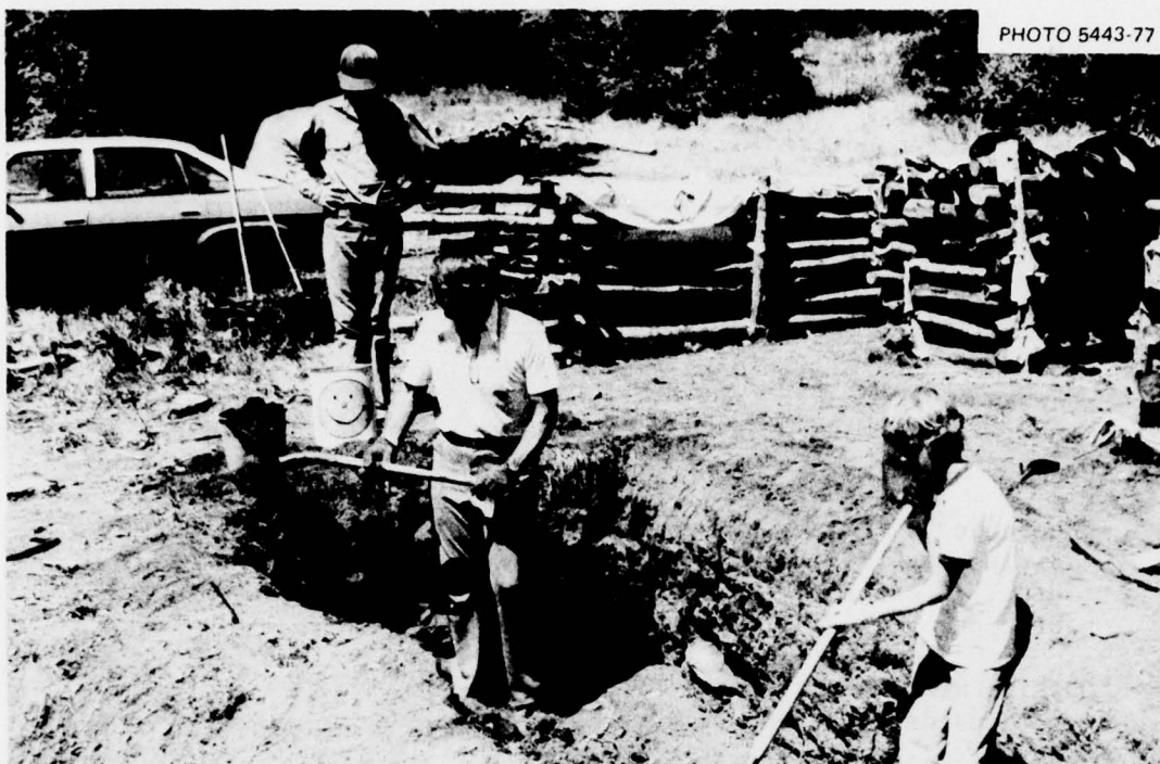
Fig. 4.22. This family, who constructed a Crib-Walled Shelter, discovered that in order to fill the cribs and cover the roof, this aboveground shelter required more digging than many trench-type shelters.
