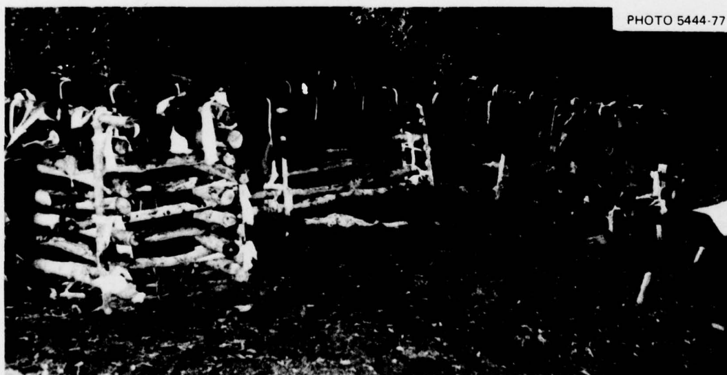
Fig. 4.23. Crib walls which have been lined and are ready to be filled. Note the use of bed-sheet strips used in lieu of rope and wire.
