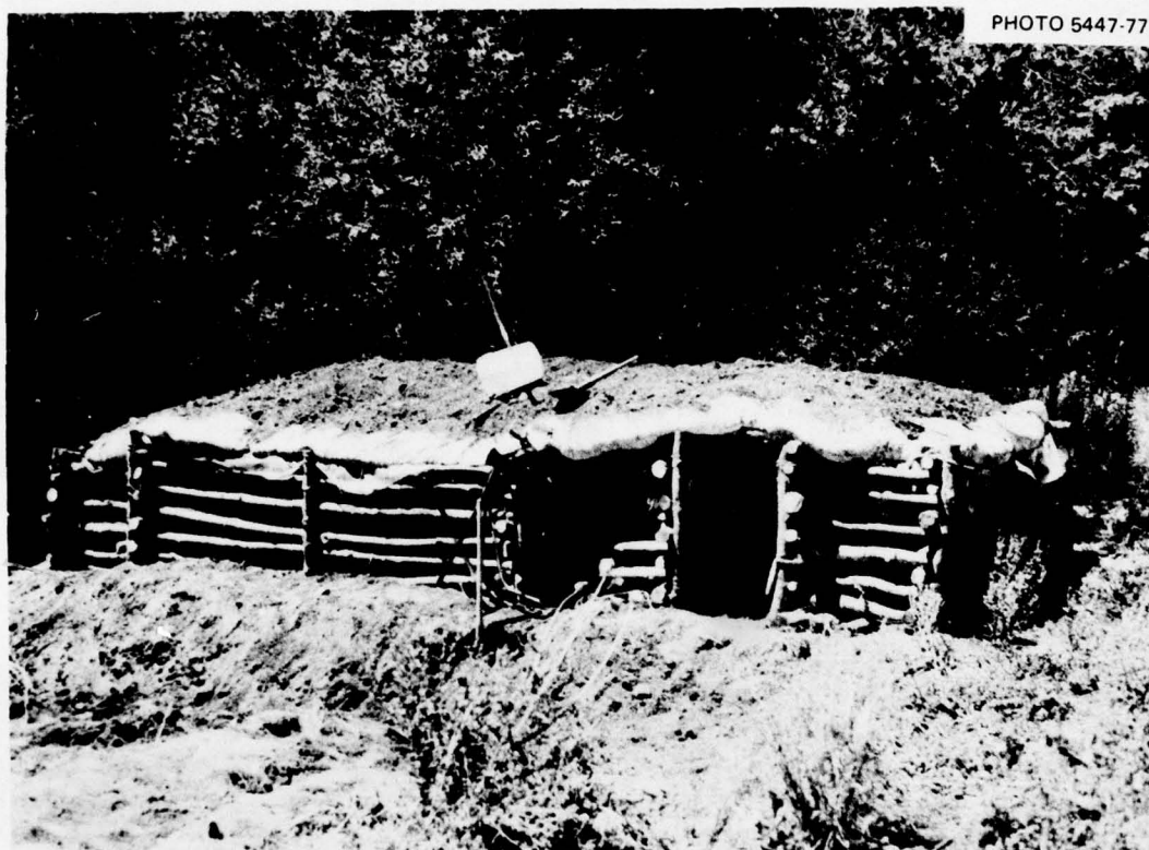
Fig. 4.26. A nearly completed Crib-Walled Shelter.
