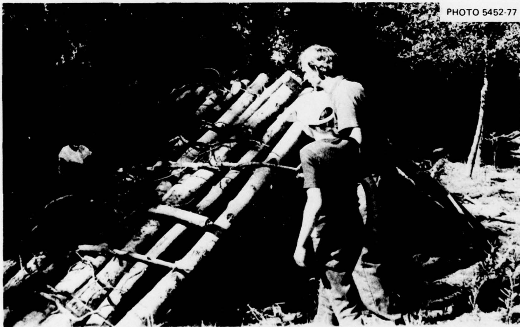
Fig. 4.29. Sticks placed horizontally. More sticks and limbs should have been used, although these few, when covered with 4-mil polyethylene, held the earth covering.
