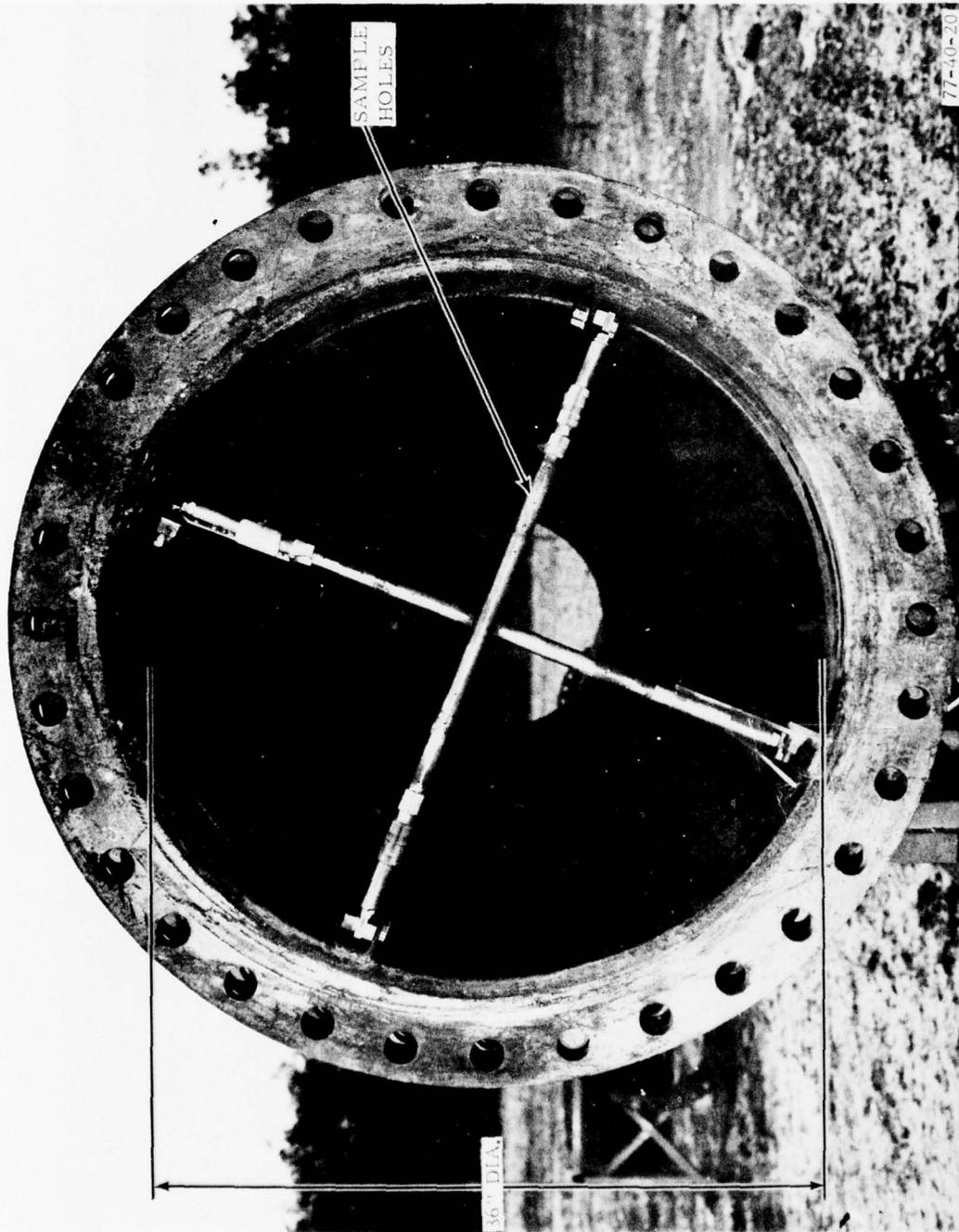
FIGURE 4. CRUCIFORM PROBE INSTALLED IN MIXER PIPE
