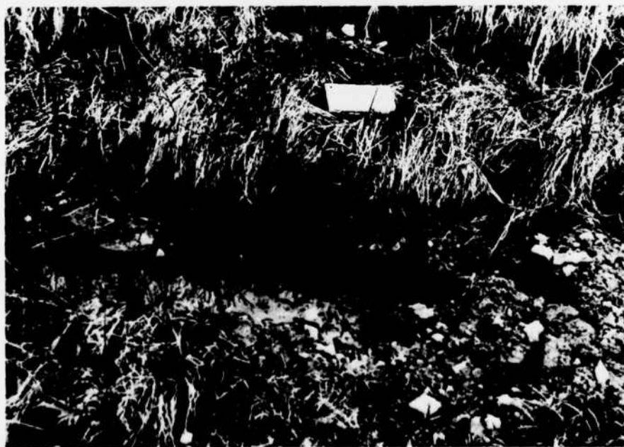
STANDING WATER ABOVE BOTTOM BERM NEAR EAST ABUTMENT
