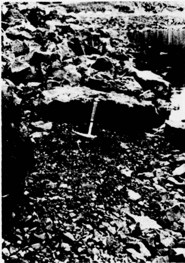
VIEW OF RIP RAPPED SLOPE SHOWING POOR GRADATION
