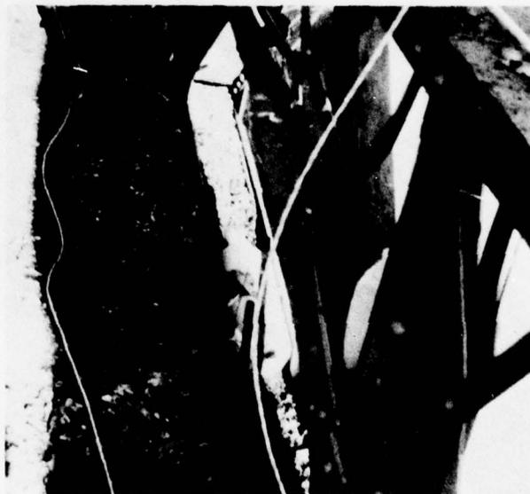
b. One 60-pound bag of slurry to cut tension member (same on both bridge trusses).
