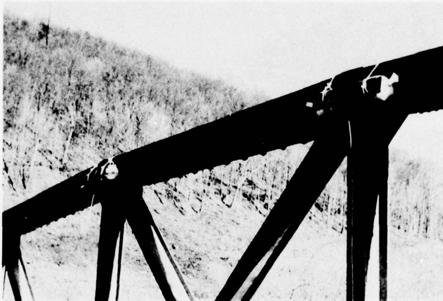
a. Two 60-pound bags of slurry to cut compression member (same on both bridge trusses).
