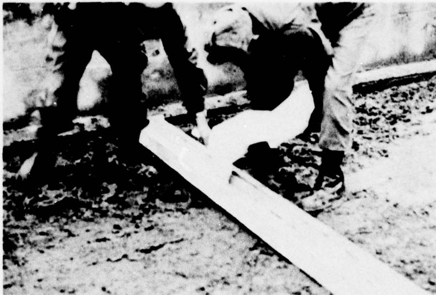
a.- Slurry being poured into 3- by 4-inch trough.
