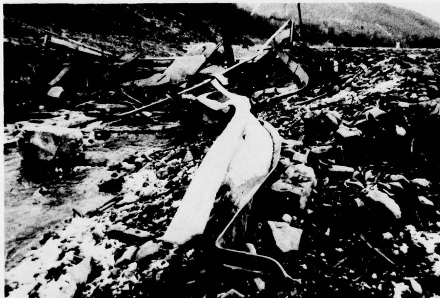
f. Twisted condition of bridge beams.
