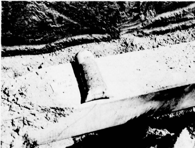
d. Concrete prestress piers with plastic bag charge containers.
