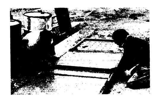
Figure 11 Casting of target slabs.
