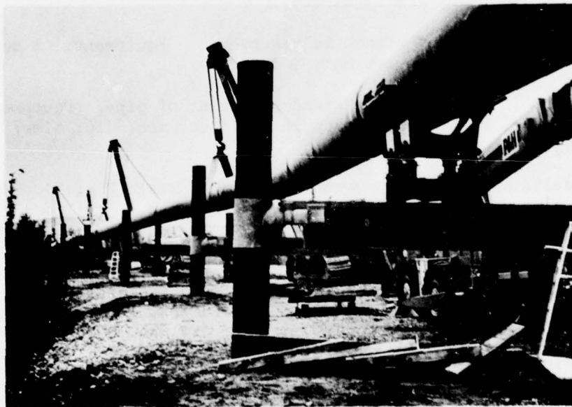
Figure 5. Vertical Support Member Supports; Installation of Pipe.
