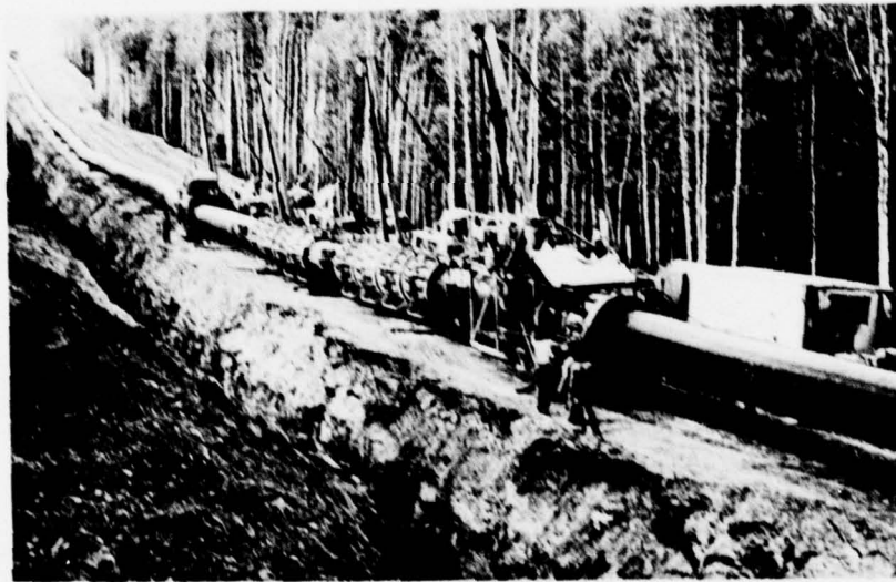
Figure 21. Pipe Taping Unit in Operation.
