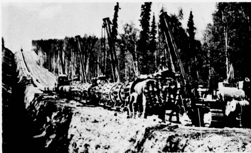
Figure 23. Taping Scene, setting up.
