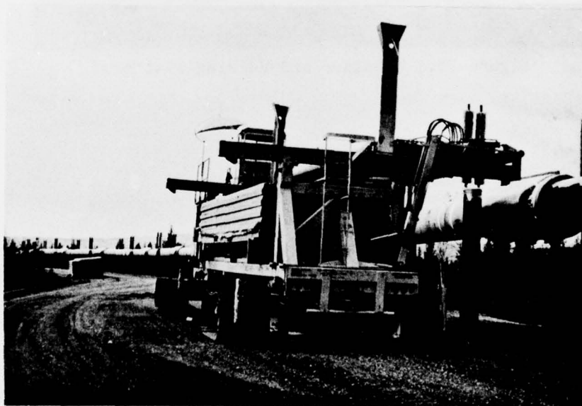
Figure 27. Stacked Panels of Folded Insulation (Background).
