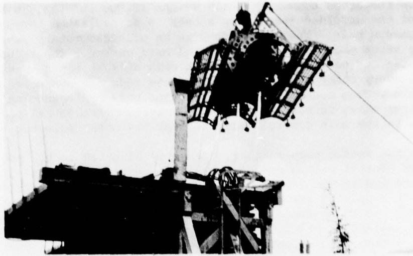
Figure 30. Panel Ready for Lifting.
