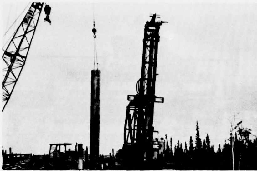
Figure 4. Vertical Support Member Installation.
