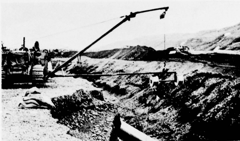
Figure 10. Cathodic Protection Installation.
