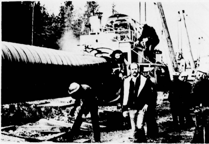
Figure 9. Pipe Taping.
