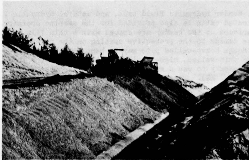
Figure 11. Trench Backfilling.
