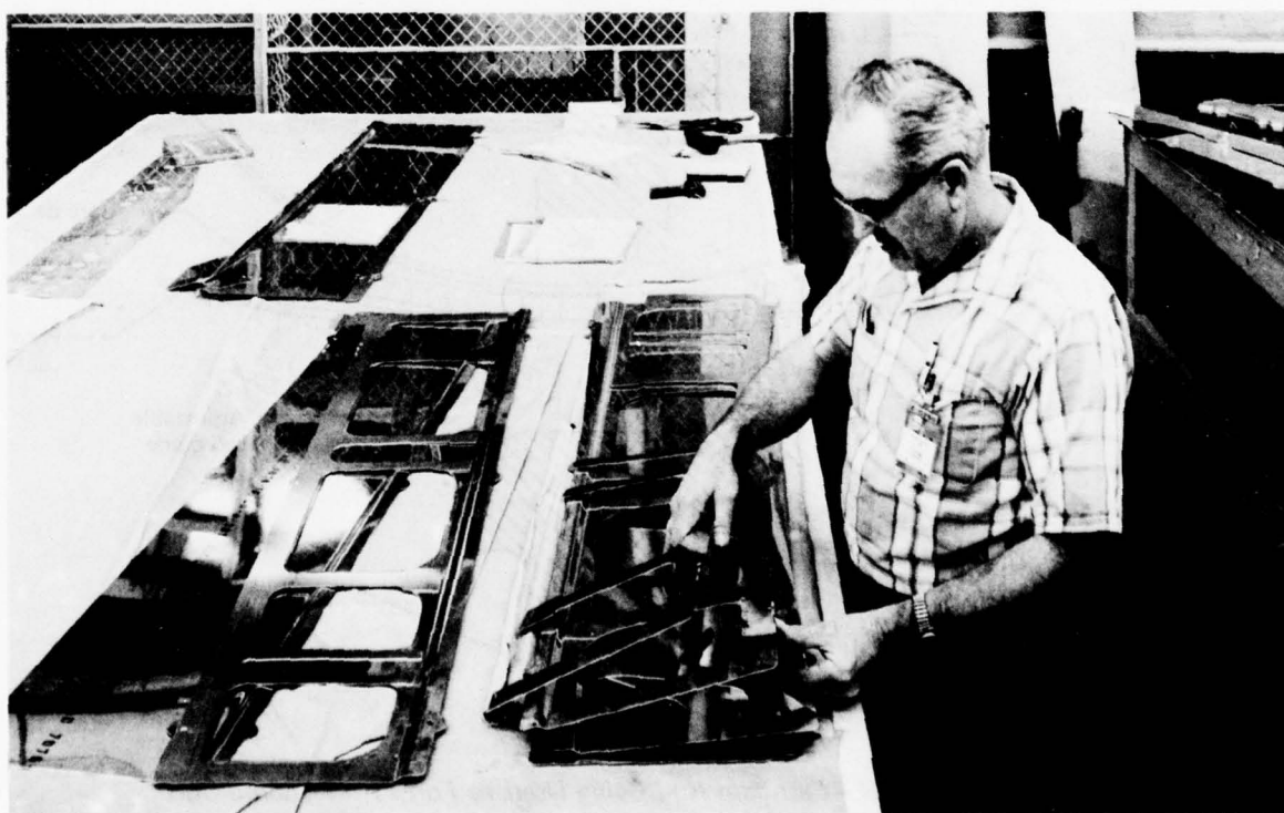
Figure 7-20.—Prefit Inspection Prior to Bonding
