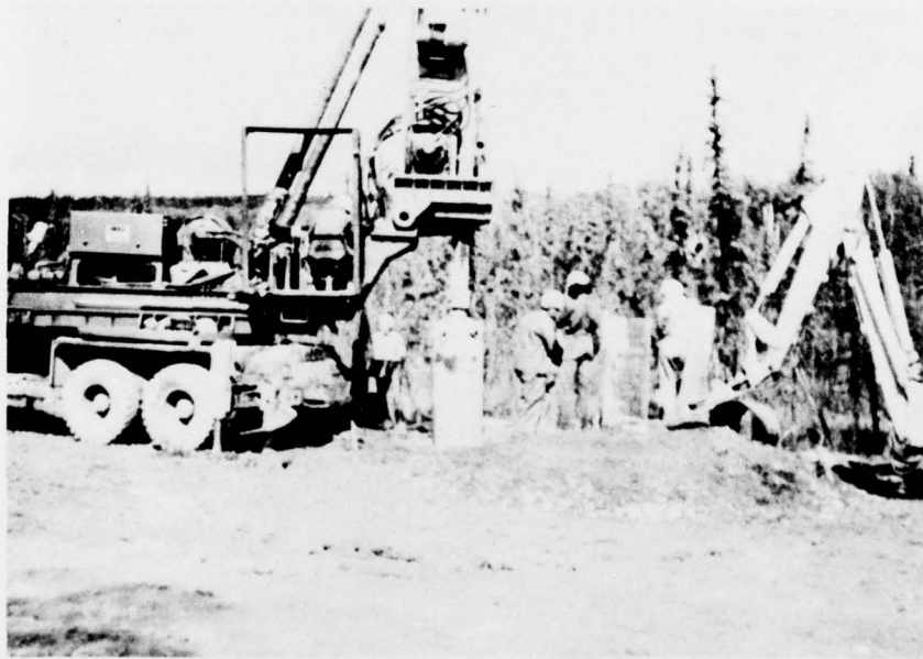
b. Installation of a casing section using a T-bar spinner.
