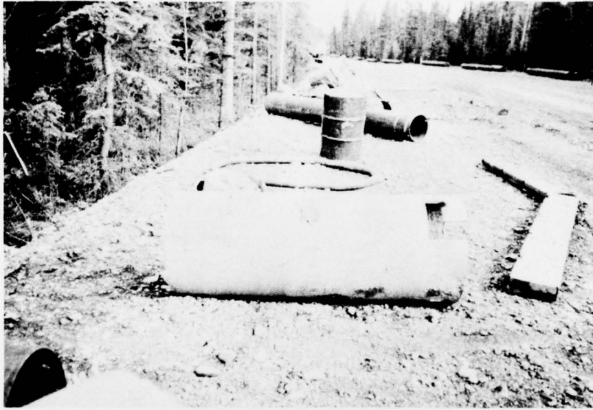
a. Casing section used with auger rigs.
