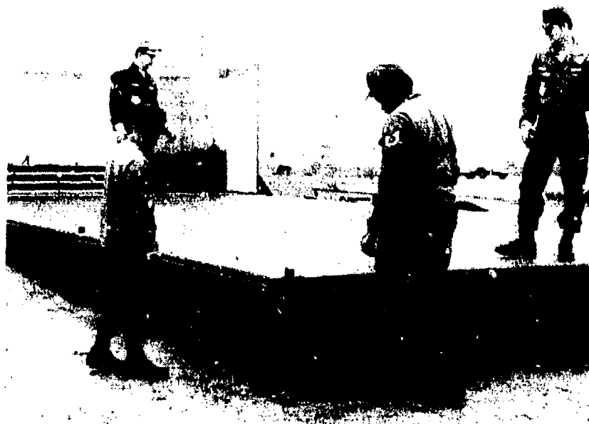
Figure A-6. Shelter Floor Levelled on 3 Percent Slope
