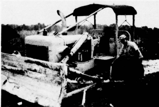
(d) Dozer easily worked itself into sinking 2 ft (operator holding 4 ft rule) in Test Area #1. Sand partly liquefied into "rolling" for c. 15 ft radius around moving dozer. (16 Sep)
