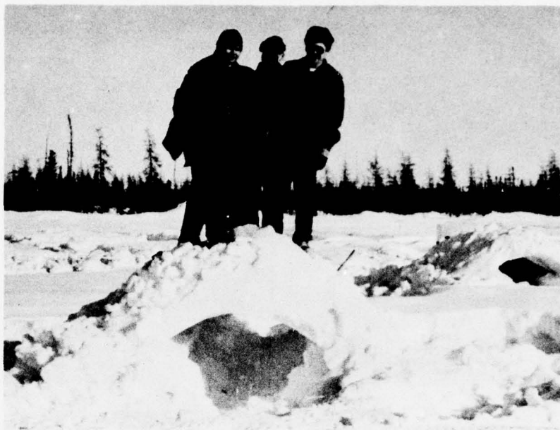
Figure 28. Snow arch after age hardening.
