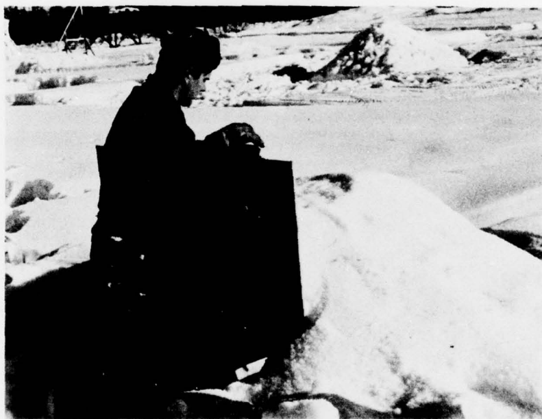
Figure 27. Snow arch form in use.
