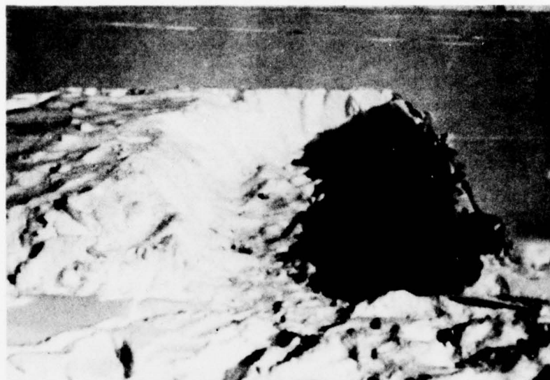
Figure 17. First hardened snow trench. Because the packed snow in front was not smooth and level, it lost some effectiveness.
