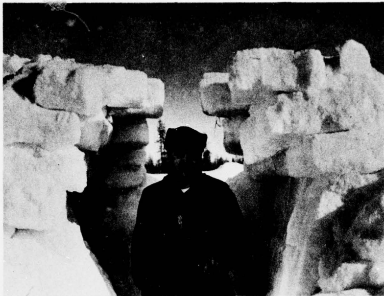
Figure 24. Partially completed snow block structure.
