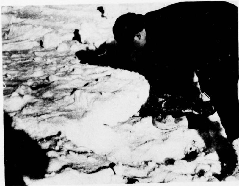
Figure 22. Mining a snow block in packed snow.
