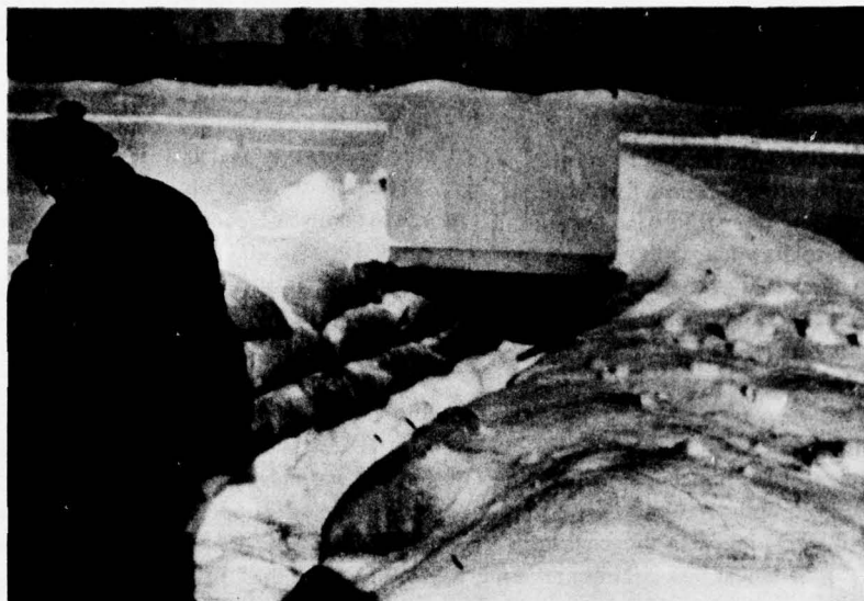
Figure 20. Snow trench revetted with snow bags.
