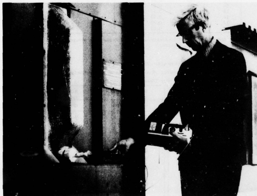
Figure 5-14. Photograph of a waveguide localizer showing one of the slot antennas.
