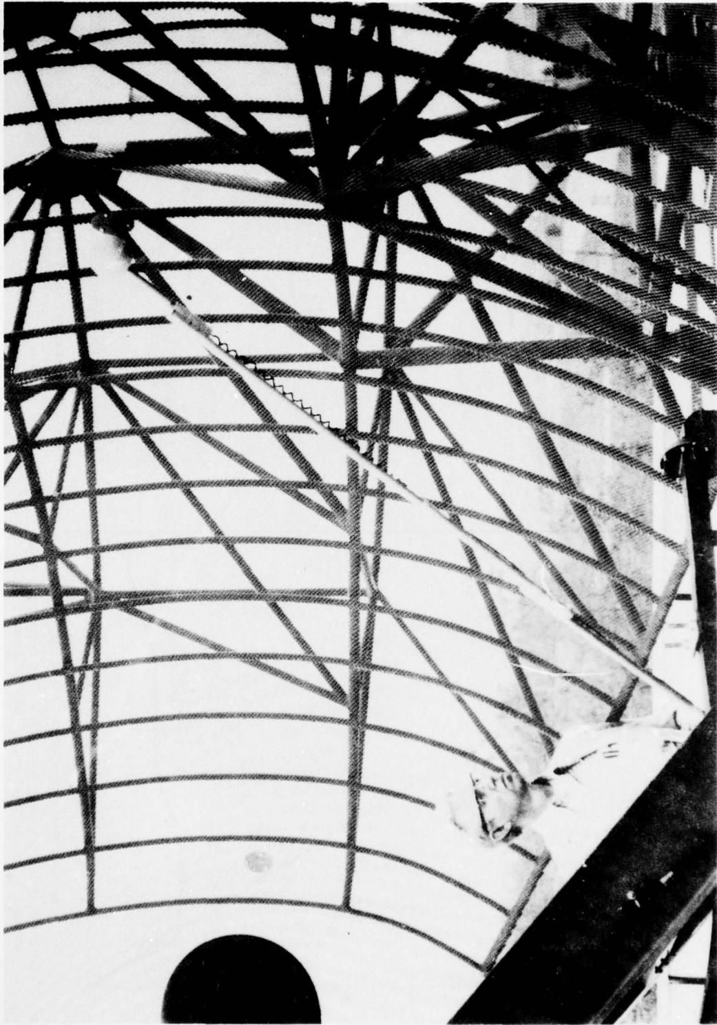
Figure 4-2. Photograph of measurements being taken in the field of an ASR antenna, closeup view of the feed and reflector screen.
