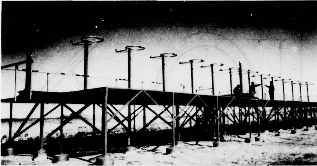
Figure 5-4. Photograph of a V-ring localizer antenna array, ILS, Denver.
