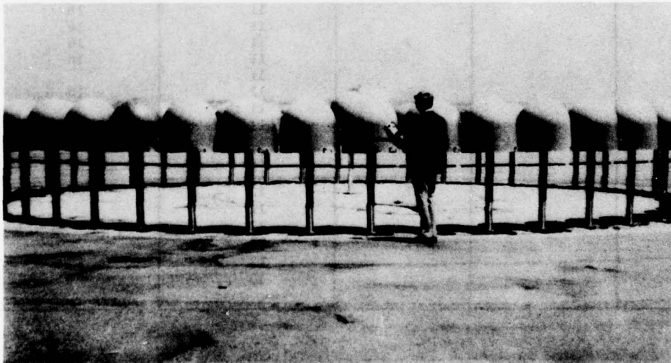
Figure 6-3. Photograph of a Doppler VOR antenna array.
