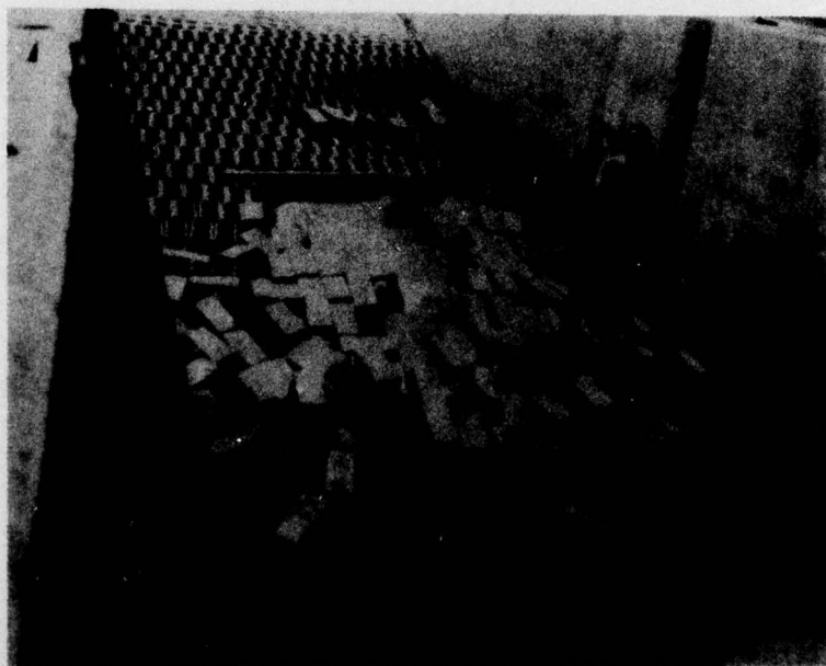
Figure 9. Damage level 4 after a 1.65 meter breaking wave. Note the displacement of the blocks and the area that has slumped.
