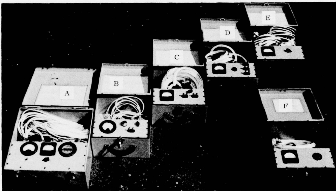
Figure A-34. Test units for helicopter and ship-or-shore equipments.
