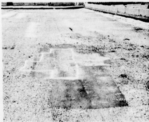
Figure 7. Daytime photograph of a patched area with a wet area outlined in white spray paint.
