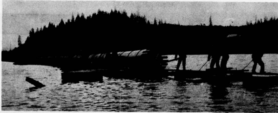
This 4,000-foot-long, 60-inch water pipe was built in the 1930's of Douglas-fir treated with a preservative salt.
