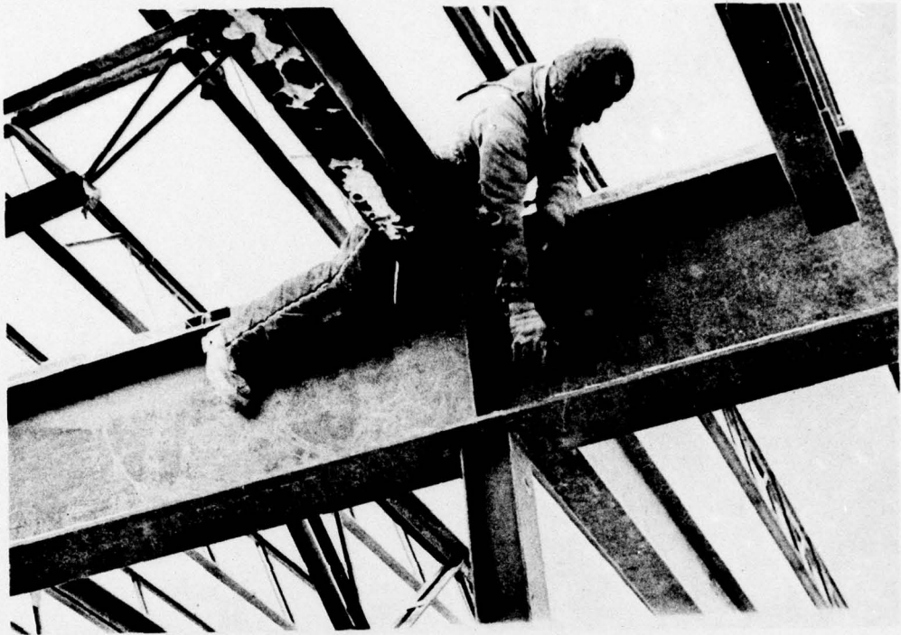
45. Ironworker installing bolts at Interior City Branch project. January 7, 1977. +14°F.
