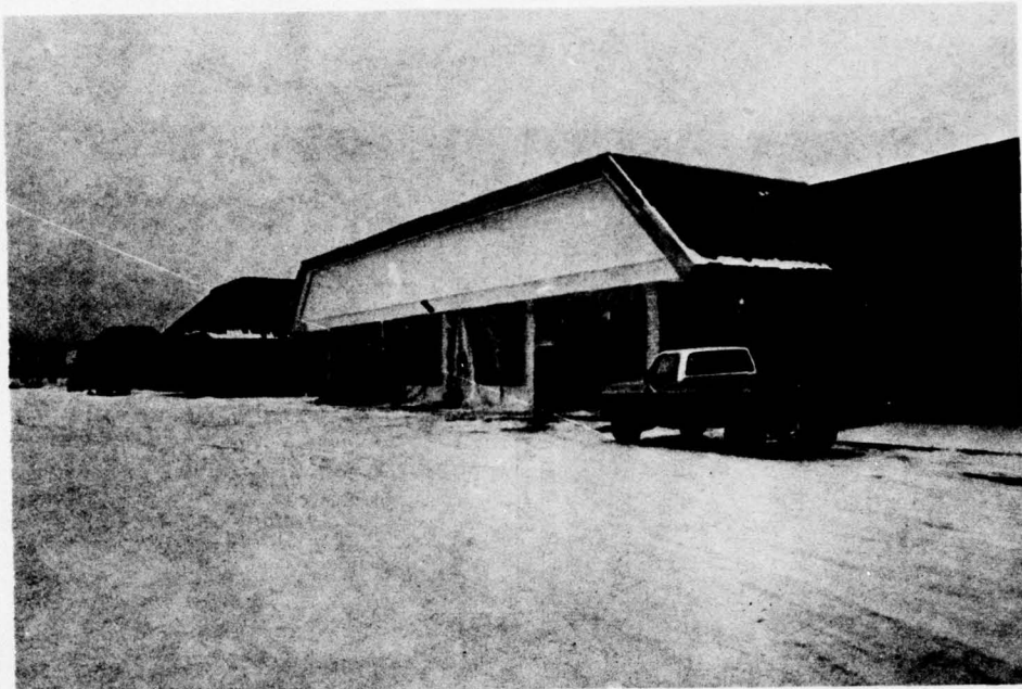
2. General View of Bentley Mall project showing permanent walls and polyethylene sheltered entrance ways. November 28, 1976. +32°F.
