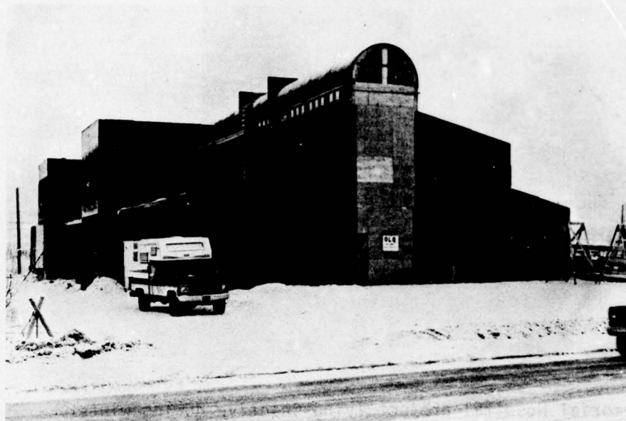
10. General view of Plywood Supply project, looking generally north. November 24, 1976. +12°F.
