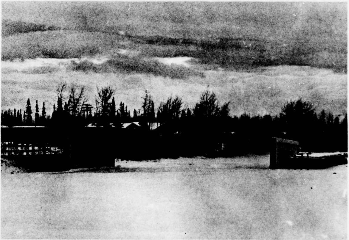
7. Steese Highway Bridge over Chena River, activities suspended over winter. November 28, 1976. 32°F.
