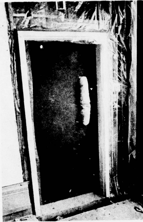
25. Partially installed door protected with insulation, Federal Building project. November 24, 1976. +12°F.
