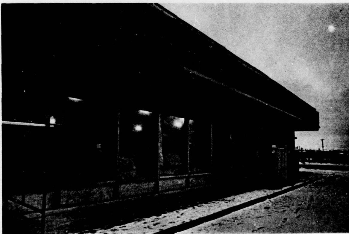
15. Temporary enclosures were window openings, Bentley Mall project. November 28, 1976. +32°F.
