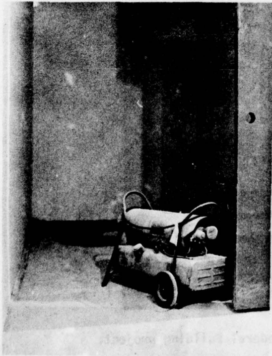
39. "Master" heater drying a damp corner at University Mall project. January 6, 1977. +4°F.
