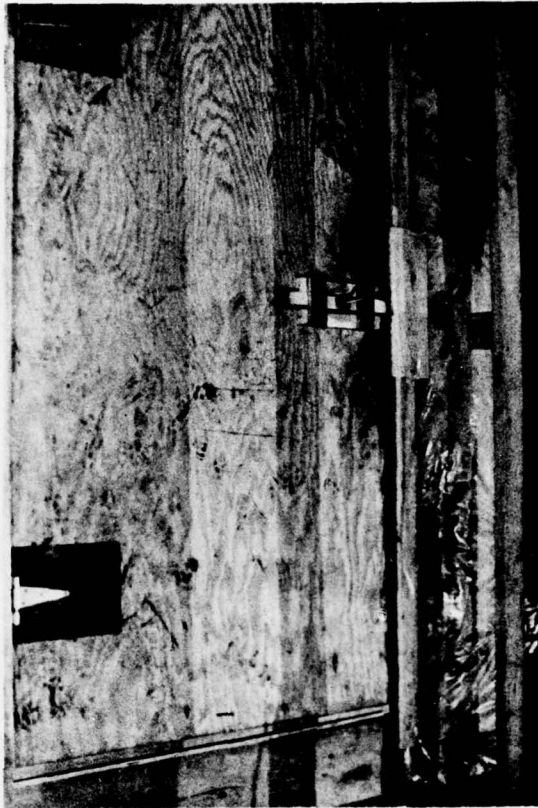
29. Temporary door at Plywood Supply project. December 30, 1976. -70°F.
