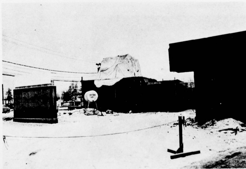
26. South and west walls of Interior City Branch project. November 28, 1976. +32°F.
