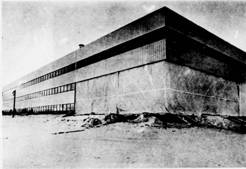
6. General View of Northeast corner of Federal Building. November 28, 1976. 32°F.
