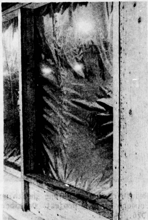
16. Close-up of temporary window coverings, Bentley Mall project. November 28, 1976. +32°F.
