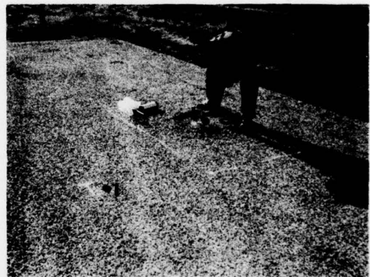
Figure 35. View of area shown in the Figure 34 thermogram.
