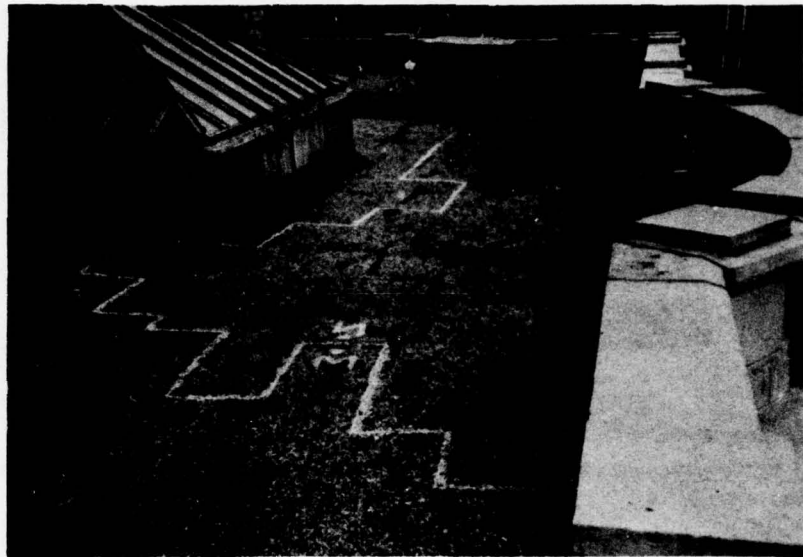
Figure 16. The area outlined in spray paint appeared darker than all other portions of the State Library roof.
