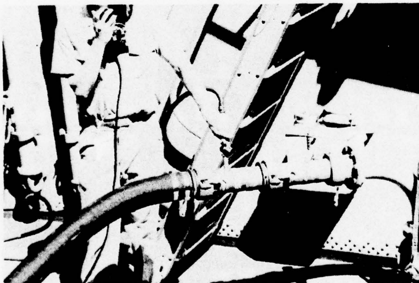
FIGURE 36 AIR BLOWDOWN FITTING
