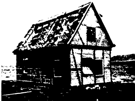
FIGURE 19 POST-SHOT VIEW OF STRUCTURE NO. 2 FROM SOUTHWEST FACHWERK SIDE
