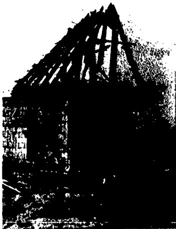
FIGURE 34 DAMAGED ROOF FRAMING ABOVE MASONRY CAVITY WALL TEST CELL STRUCTURE NO. 1
