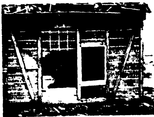
FIGURE 41 DAMAGED WEST FRONT FACHWERK WALL STRUCTURE NO. 2
