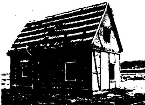
FIGURE 20 POST-SHOT VIEW OF STRUCTURE NO. 3 FROM SOUTHWEST FACHWERK SIDE
