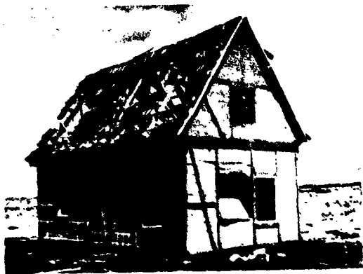
FIGURE 40 DAMAGED WEST FRONT AND SOUTH SIDE FACHWERK WALLS STRUCTURE NO. 2
