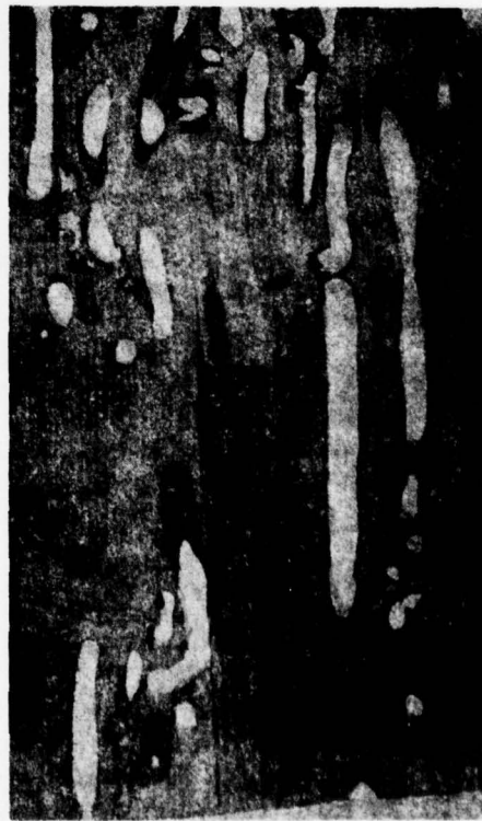
Longitudinal Section of Same Pile showing the eccentricity of the voids and extensive loss of cross-section.
