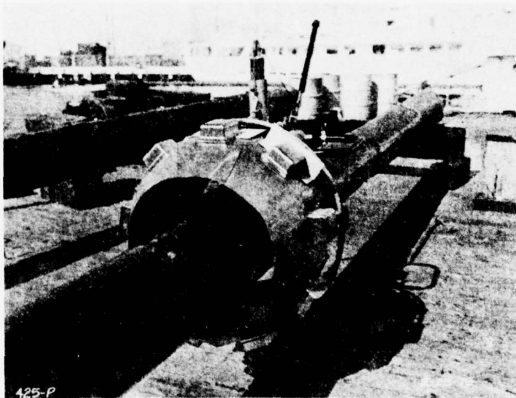
Heat Shrinking Unit shrinking 20 mil (0.5 mm) polyethylene film tightly to the pile. The Port of Los Angeles has handled and driven numerous piles without damaging the film.
