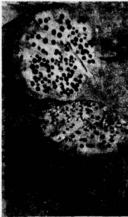
Cross-section of Above Pile showing heavy Teredine damage and loss of cross-section.
