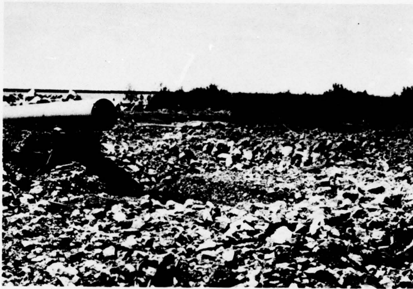
Figure 11. Outlet pipe at the Small Boat Harbor site in Buffalo
