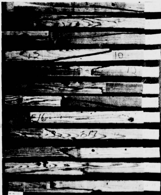
Figure 9.—Some tension laminations from beams which failed through portions of a finger joint and also through either slope of grain or grain deviations nearby; 17 beams failed in this manner. (M 143 731)
