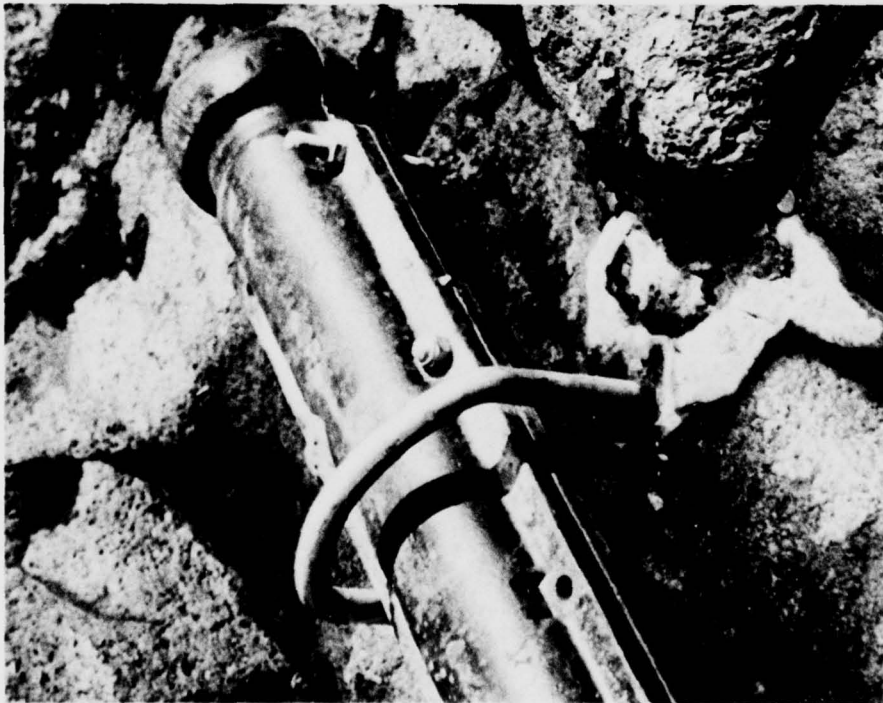
Figure 3. Grouted U-rod.
