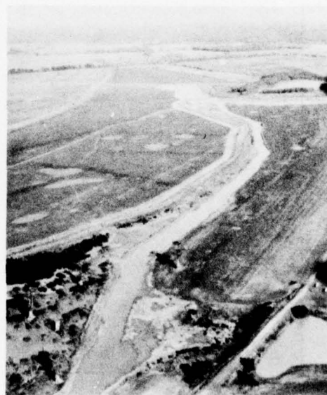
b. Drainage and irrigation canals
