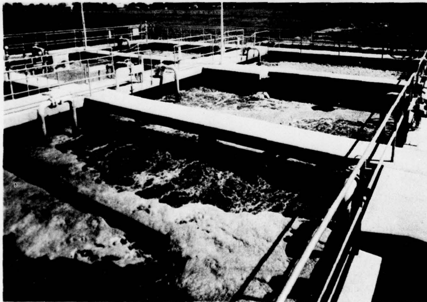
b. Activated sludge tank.
