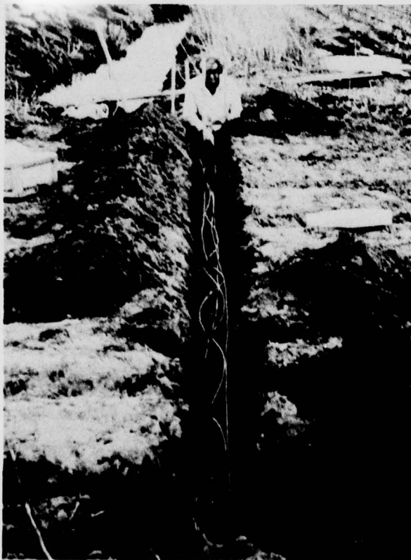
b. Installing soil solution sampling at Quincy.
