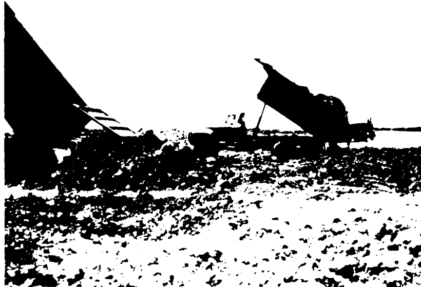
Figure 61. Trucks dumping fill material
