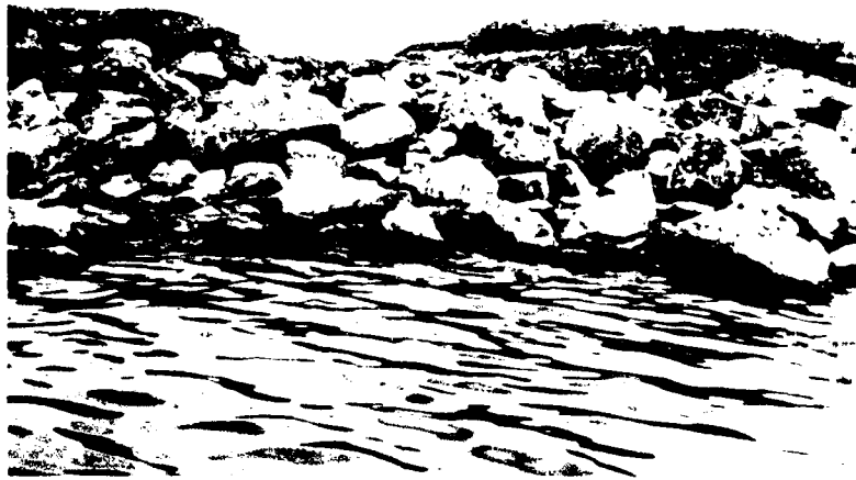
Figure 29. Damage to dike caused by overtopping
