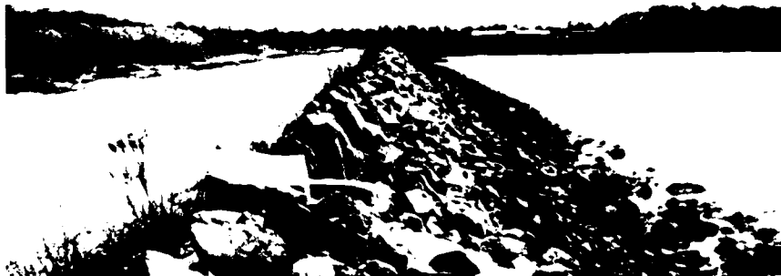
Figure 47. Typical riprap slope protection
