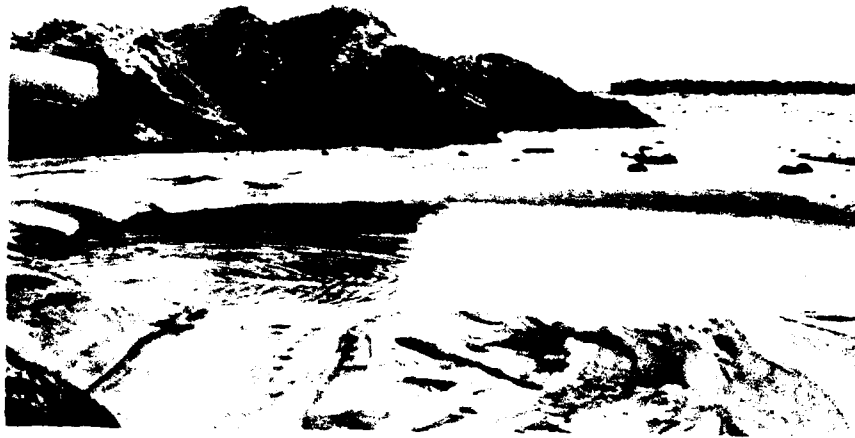
Figure 27. Depression at discharge point formed by impact of pumped material
