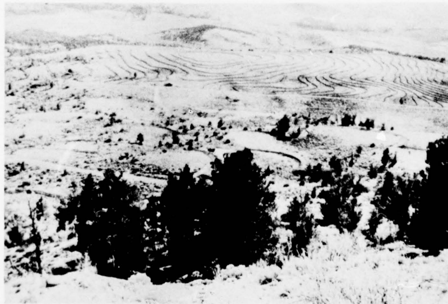
Trenching and furrowing on the National Forest to control sediment movement and runoff.
