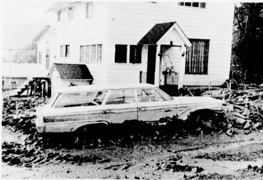
Flood damage at Telluride, Colorado from 31 July 1969 cloudburst storm on Cornet Creek, a San Miguel River tributary.
