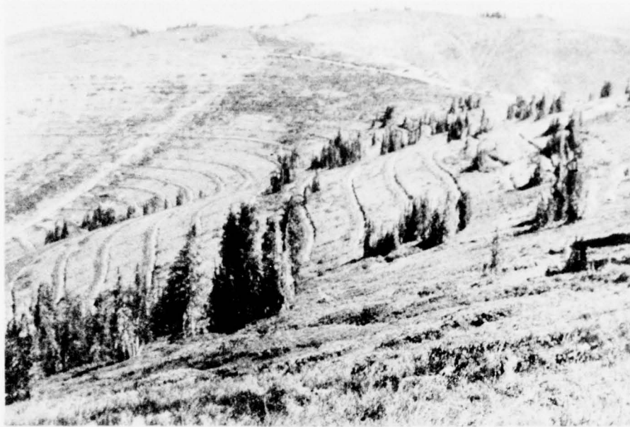
Terracing to reduce sediment yield and runoff on steep mountain slopes.
