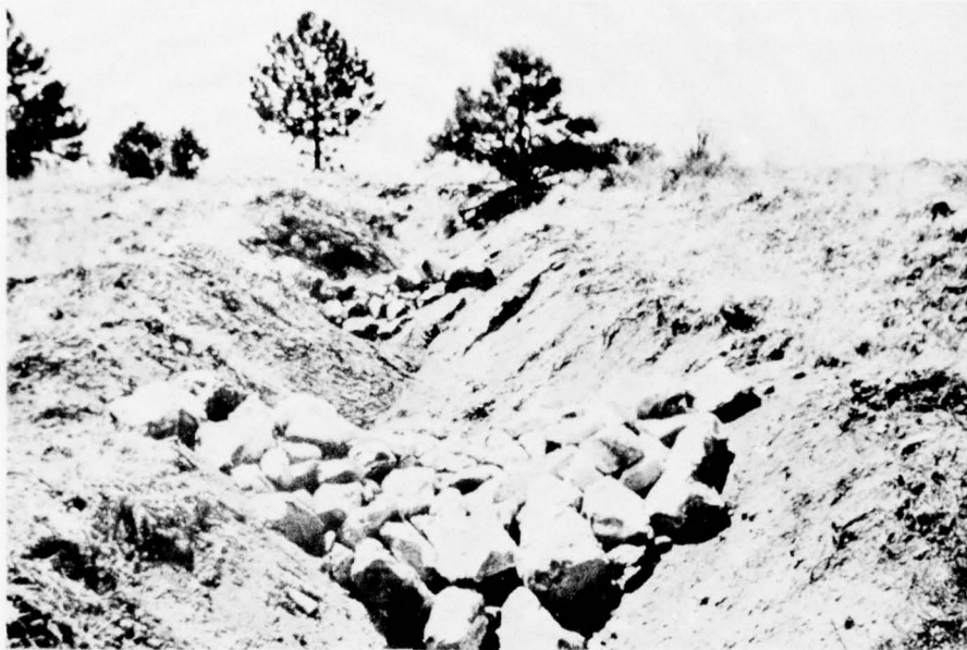
Rock check dam for control of gully erosion in watershed areas.
