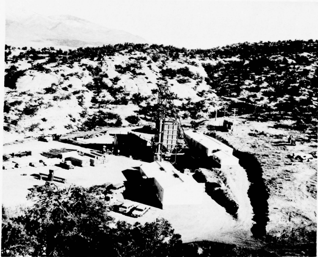
Surface plant of a typical medium-sized uranium mine in the Four Corners area.
