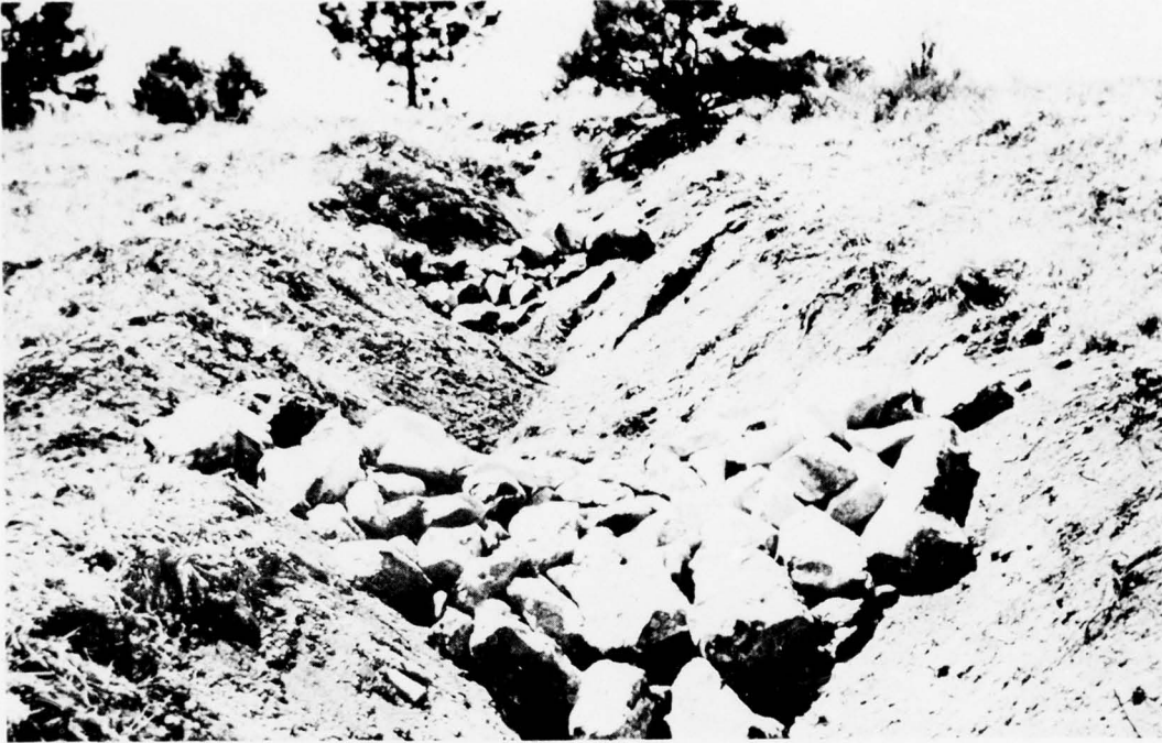
Rock check dam for control of gully erosion in watershed areas.
