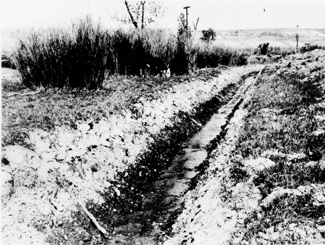
Open ditch drain newly constructed in irrigated lands in Colorado to relieve waterlogged condition and improve crop production.
