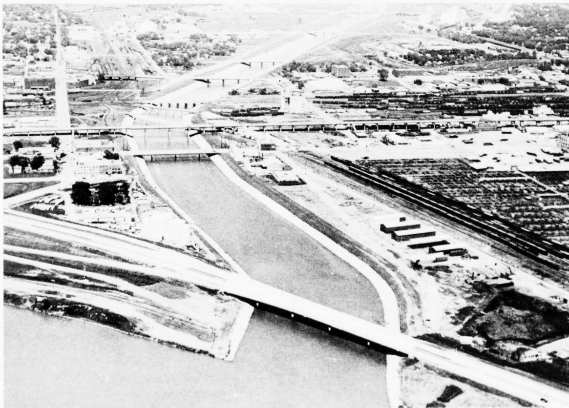
Flood Control Projects Protect Developed Areas. Floyd River at Sioux City, Iowa, Middle Missouri Subregion
