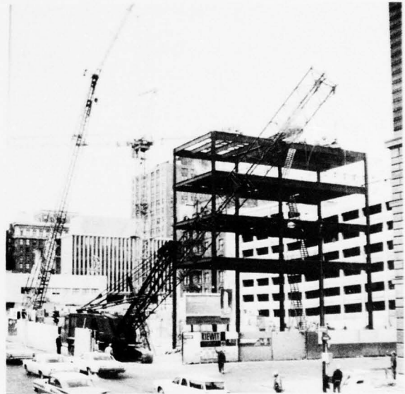
Early Construction on the Woodman Tower. Omaha, Nebraska, Belies Its 30 Story, 460-Foot Height, and 370,000 Sq. Ft. of Floor Space.
