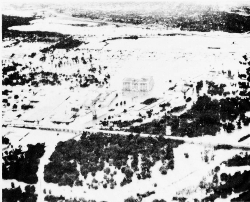
1949 FLOOD ON THE CLEAR FORK AT FORT WORTH
