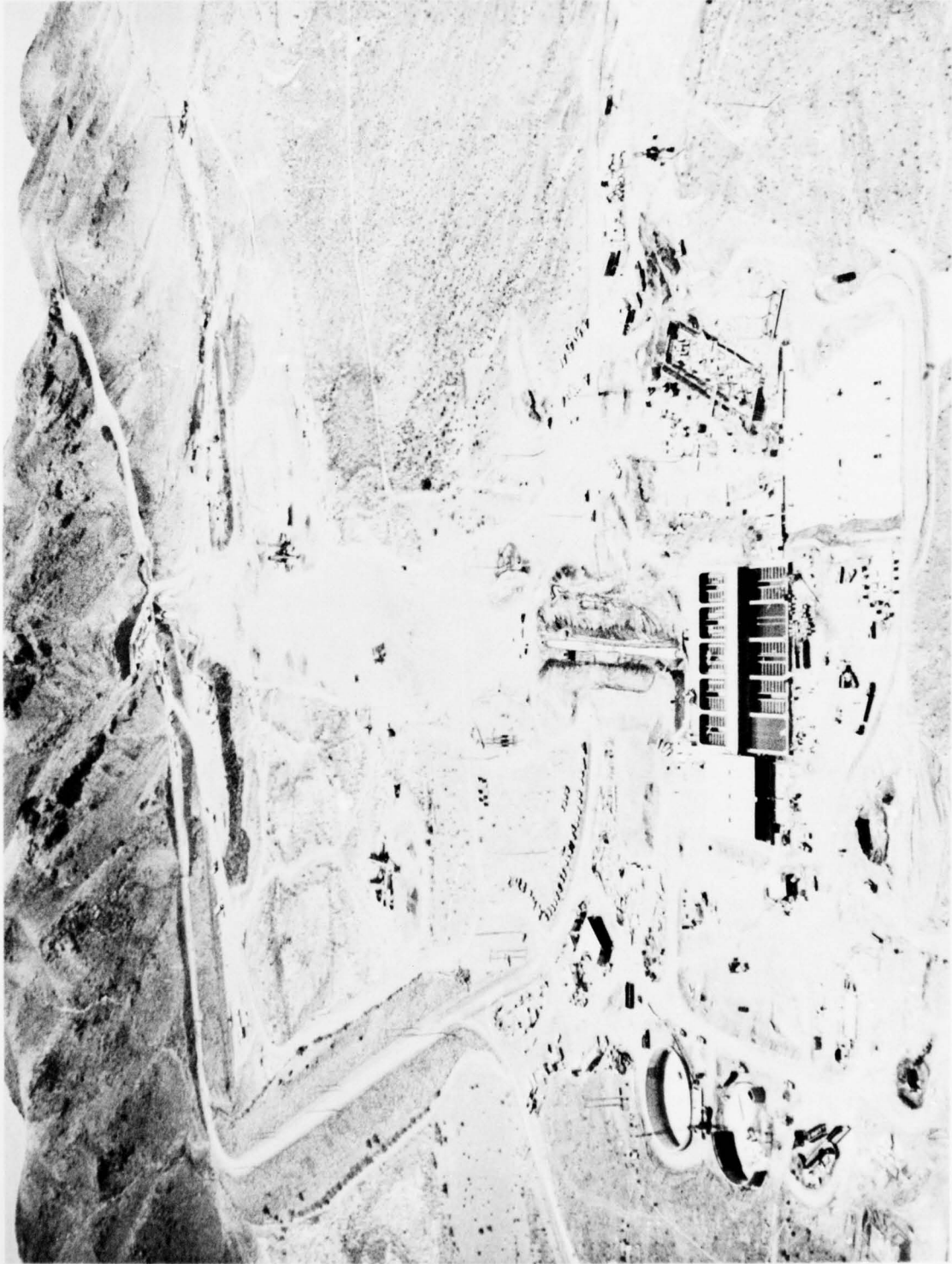
Headworks of the Southern Nevada Water Project, a part of the early action program, will supply water to the Las Vegas metropolitan area
