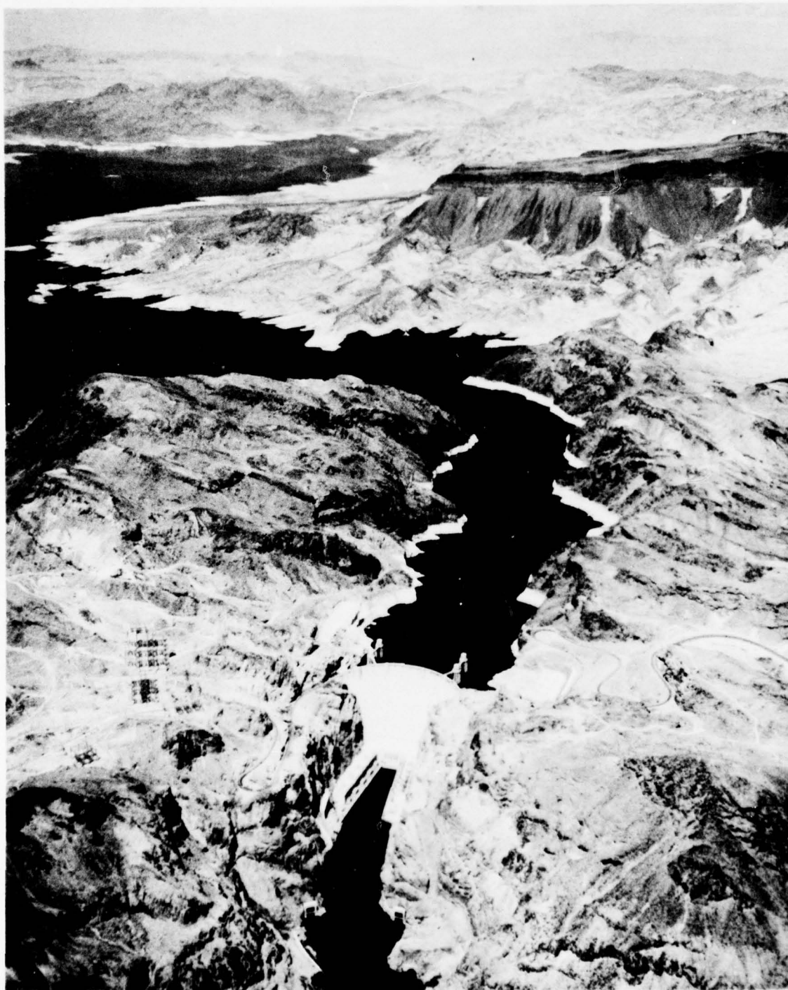
Hoover Dam and Lake Mead exemplify the concept of multipurpose use of stored water including: flood control; power generation; irrigation; recreation; fish and wildlife and other uses
