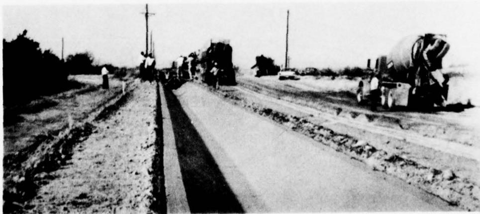
Lining of distribution ditches is necessary for increased efficiency of irrigation water use.
