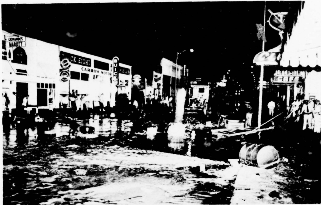
Photo 2. Damage to the business section of Globe, Arizona, from flood of July 1954. (Photo by Norman's Studio, Globe, Arizona)
