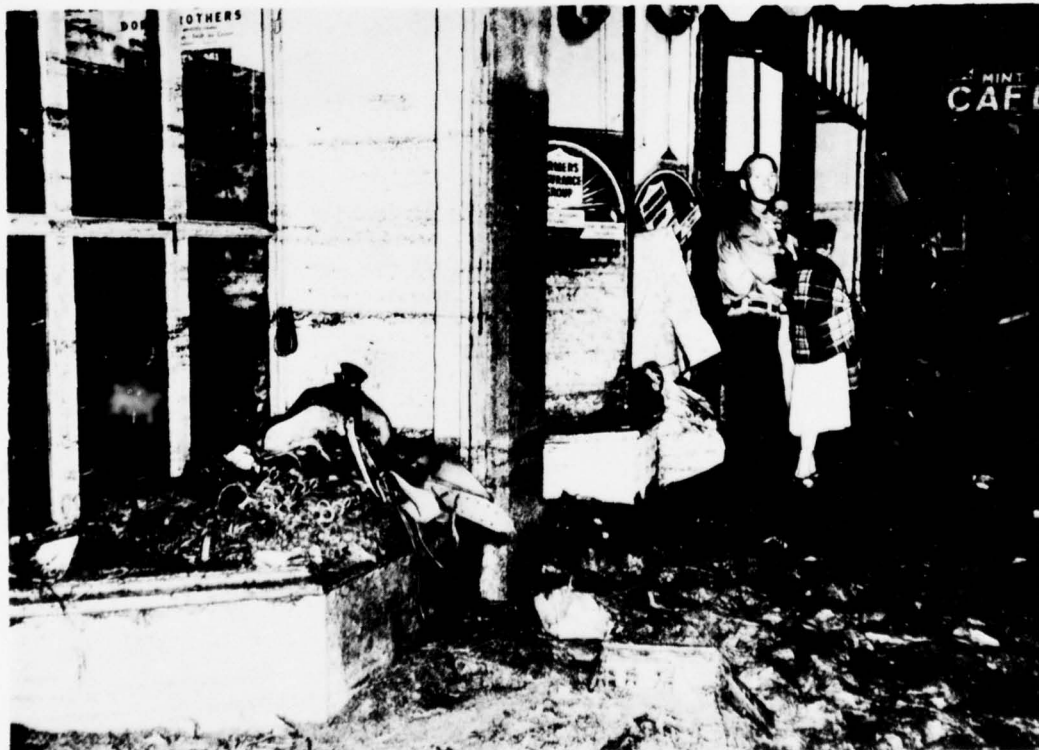
Photo 3. Typical damage to stores along North Broad Street in Globe, Arizona, from flood of July 1954. (Photo by Norman's Studio, Globe, Arizona)
