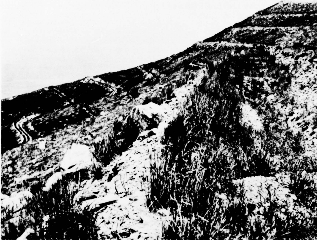
Photo 4. Contour trenches installed for flood prevention. (U.S. Forest Service photo.)
