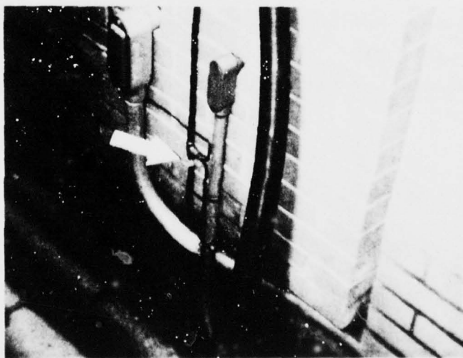
Figure 6. Down Conductor Cross Bonded to Nearby Metallic Objects.
