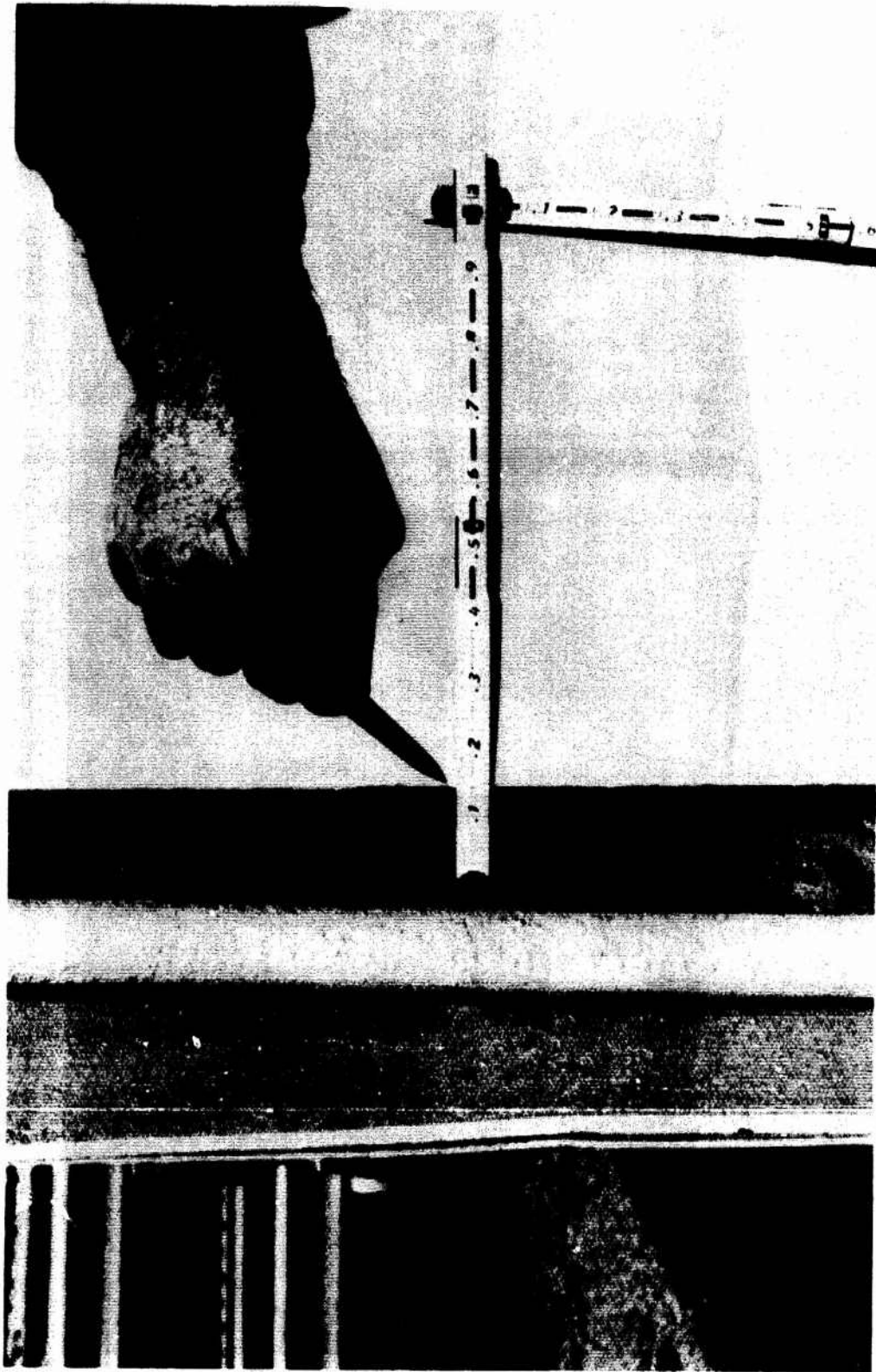
Figure 11. Gap between the generator frame and end of the generator blade.
