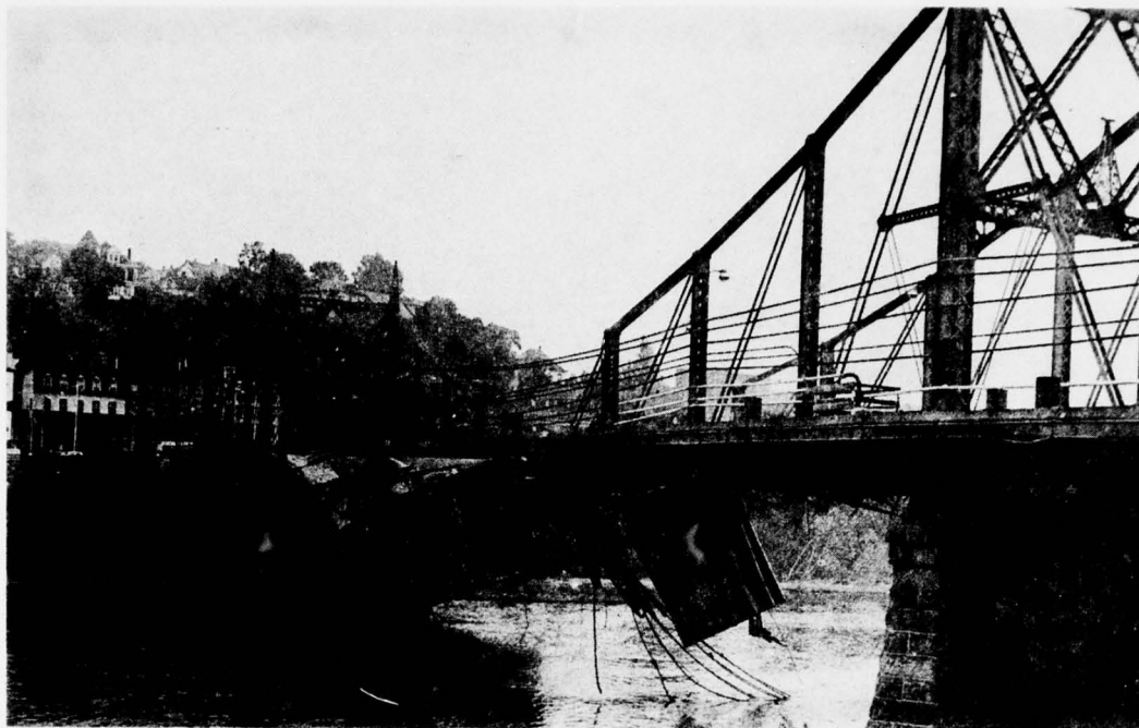
Figure 1. - Delaware River at Easton, Pa. - Phillipsburg, N. J. - Highway bridge destroyed by flood of August 1955.
