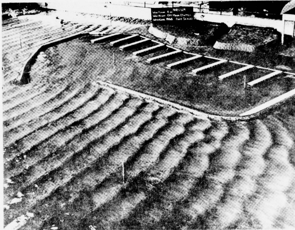
2. This 1:120 model of Napier Harbour, New Zealand, incorporating one of several proposed improvements, was built in one of the four large wave basins available at the Station for coastal engineering studies.
