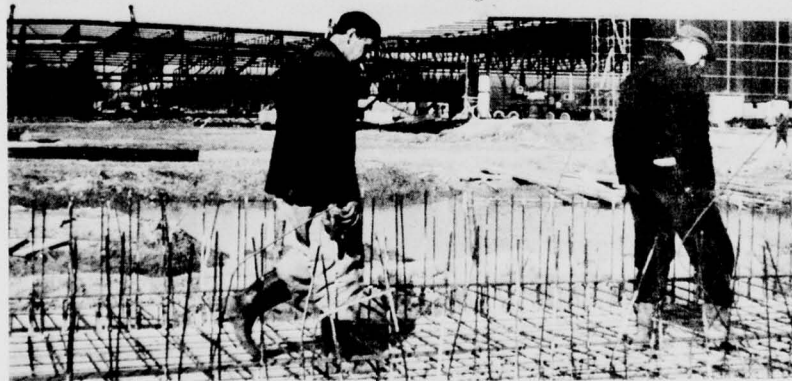
Fig. 7. Six-acre model shelter under construction at Laboratory De Voorst
